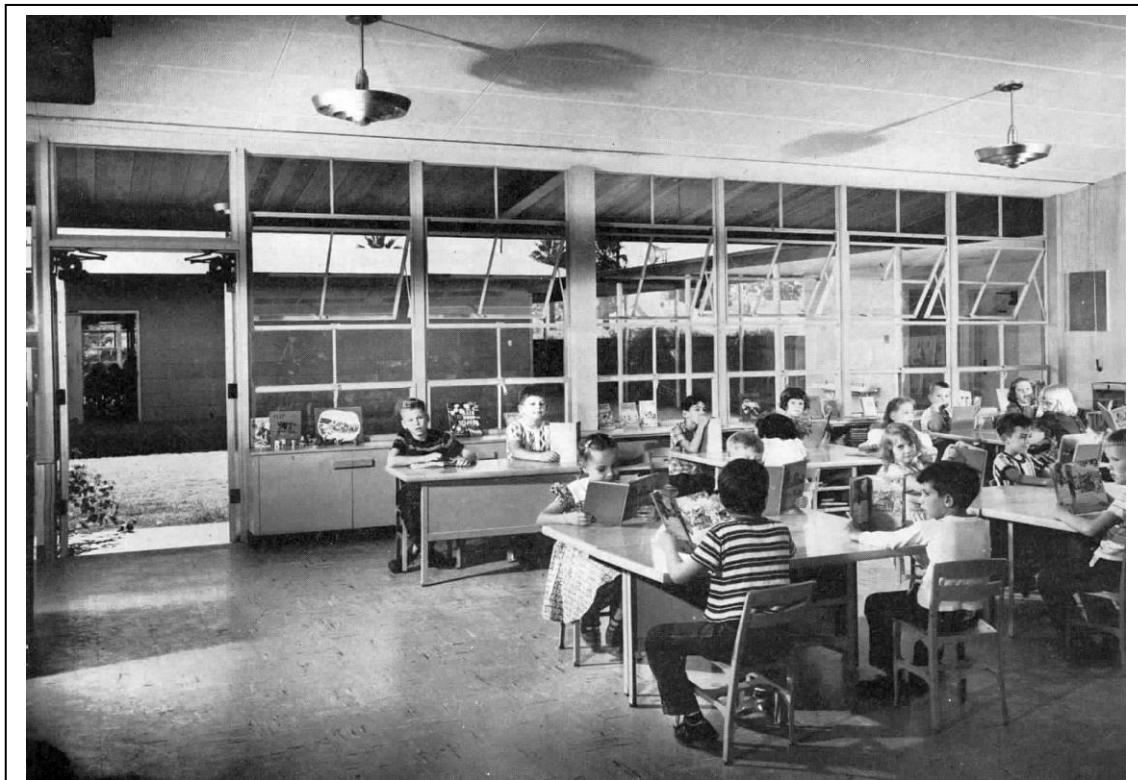
Figure 1: Monterey Park School, 1951 Source: Progressive Architecture , August 1951, p. 74
