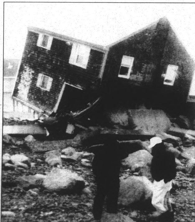
Neighbors inspect damage of an oceanfront house that was knocked free by wind and tide along Peggotty Beach in Scituate, Mass., Thursday.
