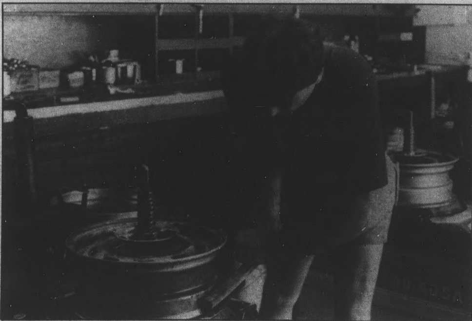
An employee of Discount Tires in Tempe cleans a corroded rim before mounting a new tire.
