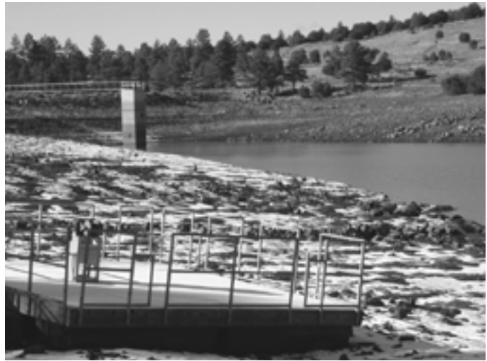
KAIBAB LAKE IN DROUGHT Extremely low water levels in Kaibab Lake, a water source for Williams, exposed most of the water intake structure (upper left) and stranded a floating dock (lower left).
