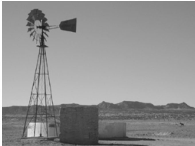
WINDMILL NEAR COPPERMINE In drought conditions, this windmill represents one of the few potential water sources for livestock on the Coppermine Chapter of the western Navajo Reservation.
