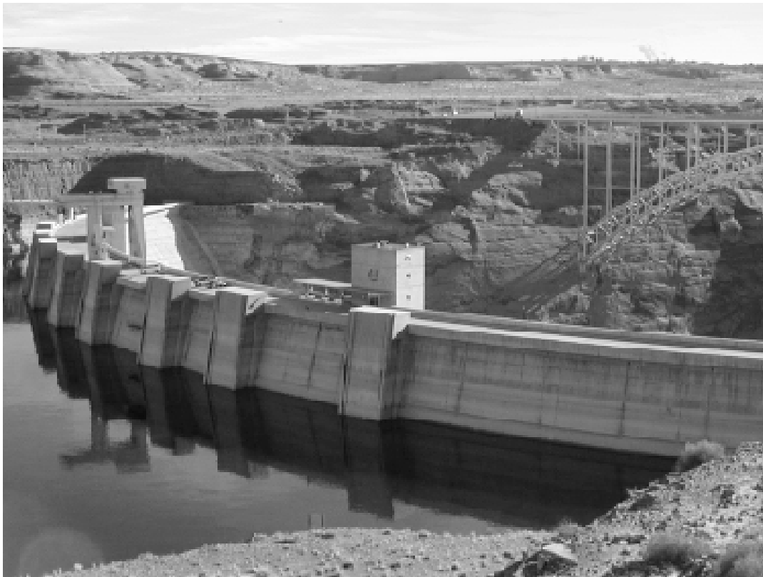
THE RESERVOIR Under a proposed pipeline, Colorado River water backed up by Glen Canyon Dam would be diverted to several north-central Arizona communities, including Page (on horizon, upper right).
