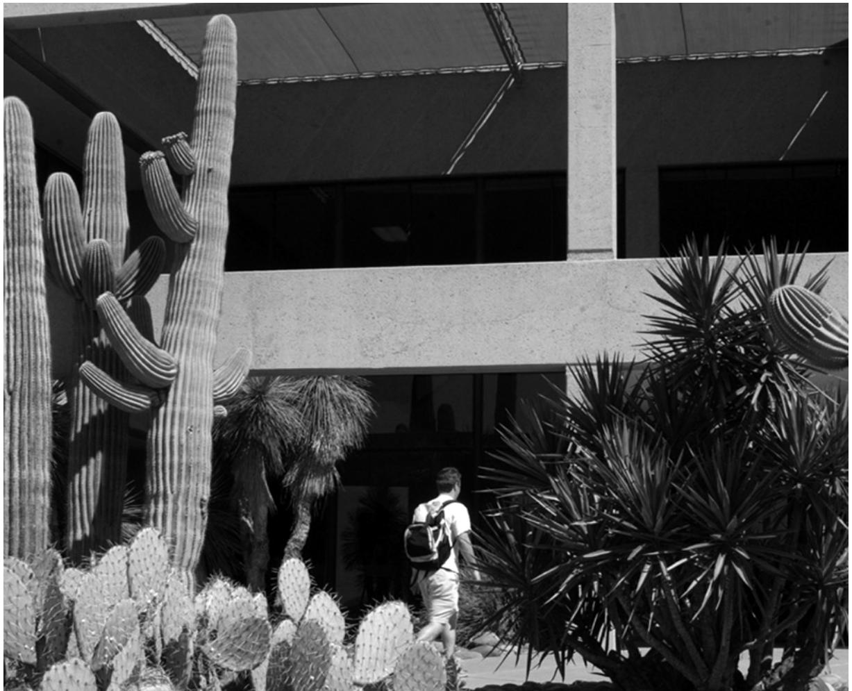
The Flight Simulator Building is a prominent facility for Polytechnic campus Master of Technology programs.
