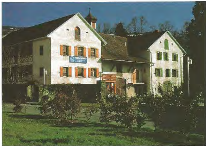
▲ The Thunderbird facility in Archamps, France is located in the International Business Park close to the Swiss/French border near Geneva.
