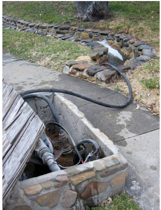
Figure 10 – The 300-foot TK Bar Ranch Well #1 is shown pumping into a river-rock lined ditch. Nearby is the 500-foot TK Bar Ranch Well #2 that has artesian flow. Samples (UHA-37 and UHA-38) from both wells met all water quality standards.
