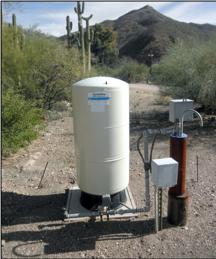
Figure 2 – A domestic well drilled in the floodplain down-gradient of the Aravaipa Canyon Wilderness Area.
