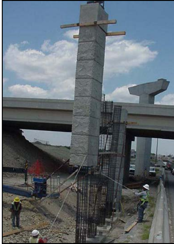
Figure 26. Lifting Precast Column Shell into Place, SB 340 over IH-35. (Wolf 2005.)
