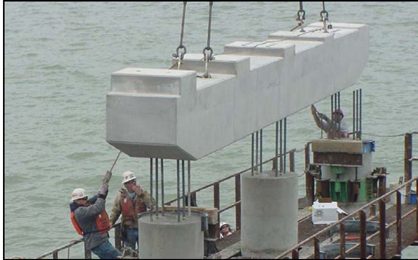
Figure 23. Placement of Precast Bent Cap on Lake Ray Hubbard Bridge. (FHWA 2009.)
