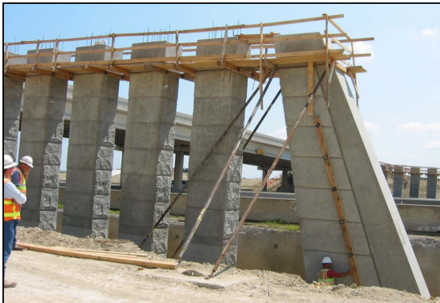
Figure 27. Precast Column Shells Before Core Filling on SB 340 over IH-35. (Wolf 2005.)
