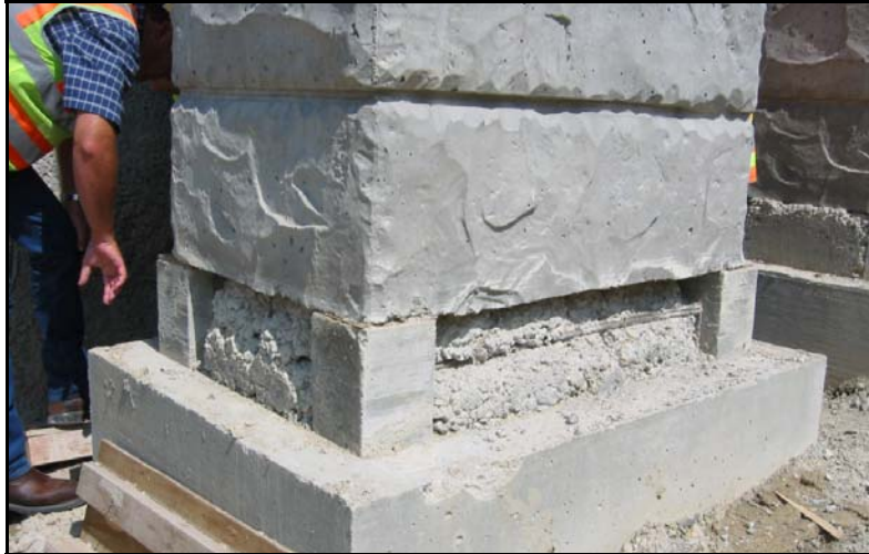
Figure 28. Base of Precast Column Shell After Core Concrete Filling. (Wolf 2005.)
