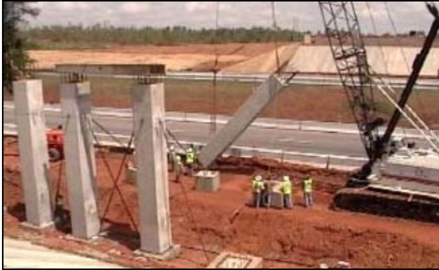
Figure 8. Erection of Precast Concrete Columns on Kia Boulevard Bridge. (FHWA 2010b.)
