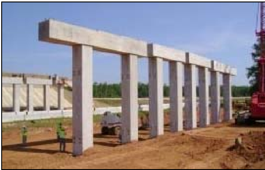
Figure 9. Completed Intermediate Bents on Kia Boulevard Bridge. (FHWA 2010b.)
