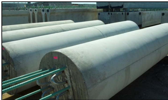
Figure 12. Precast Columns in Casting Yard on Parkview Avenue Bridge. (Photo Courtesy of MDOT)
