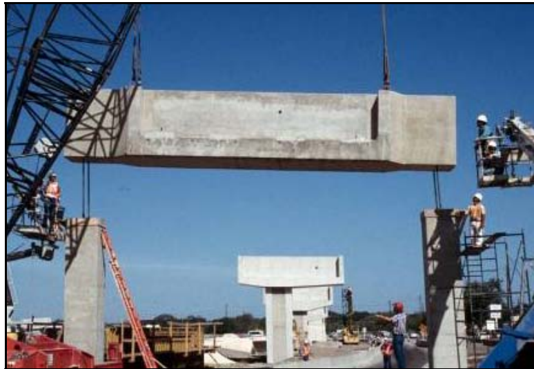
Figure 20. Precast Bent Cap Lowered into Position on Ramp E-3 Structure. (Marin 2008.)
