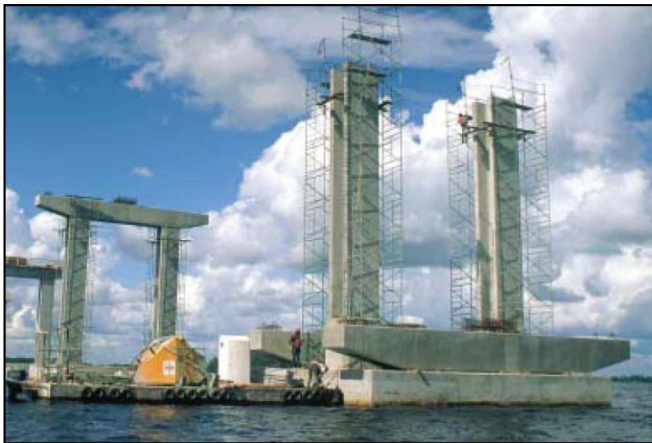
Figure 6. Erection of Precast Bents on Edison Bridge. (Ericson 2005.)
