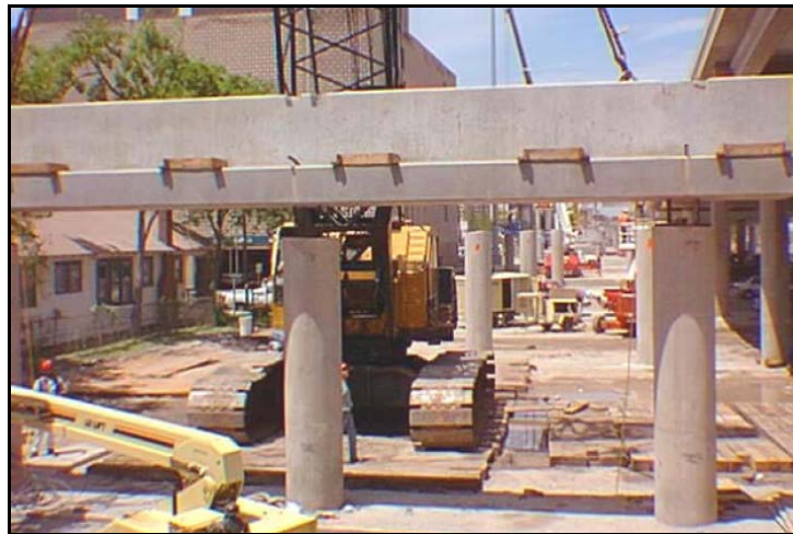
Figure 22. Precast Cap Placement on Pierce Elevated Freeway, Houston. (Wolf 2005.)
