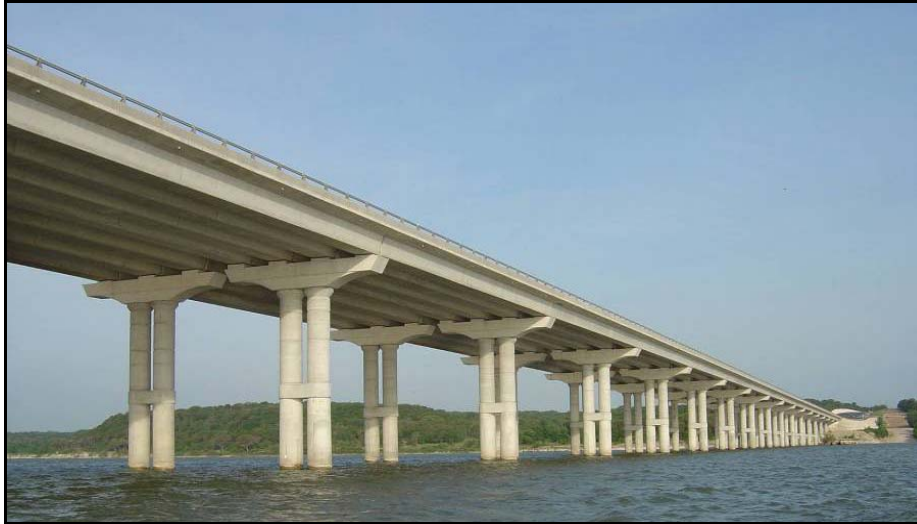
Figure 25. Completed Lake Belton Bridge. (Marin 2008.)
