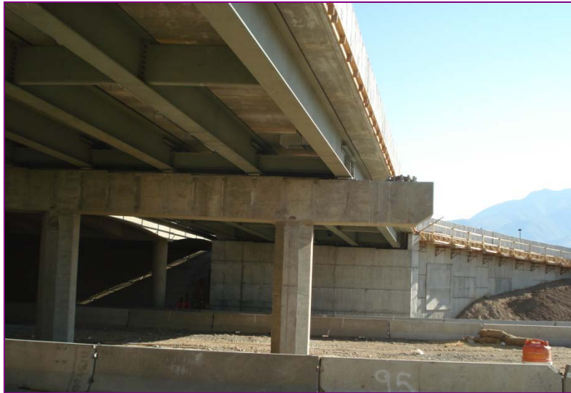
Figure 32. Riverdale Road Bridge in Utah. (Burns 2008.)
