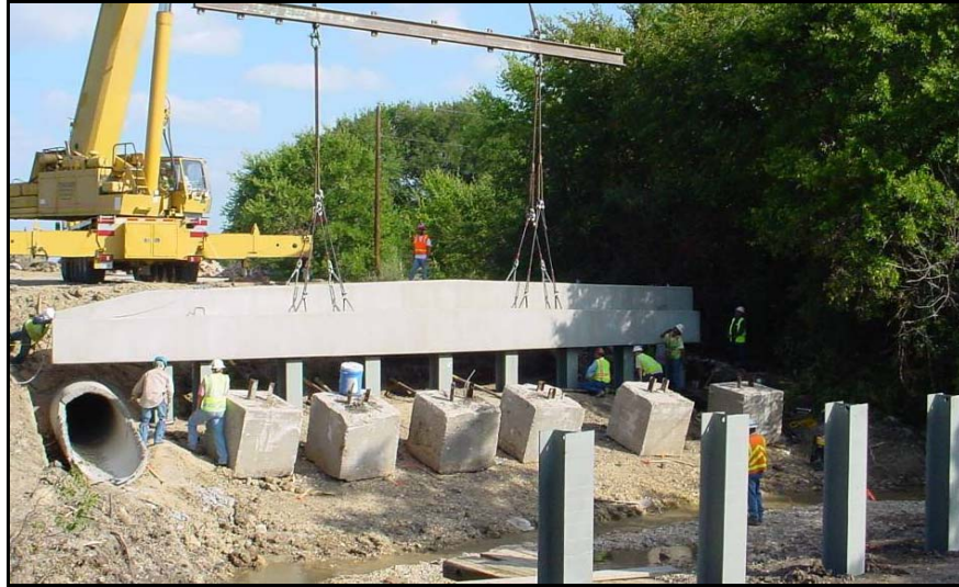
Figure 30. Installation of Precast Abutment, Cottonwood Creek Bridge. (Marin 2008.)
