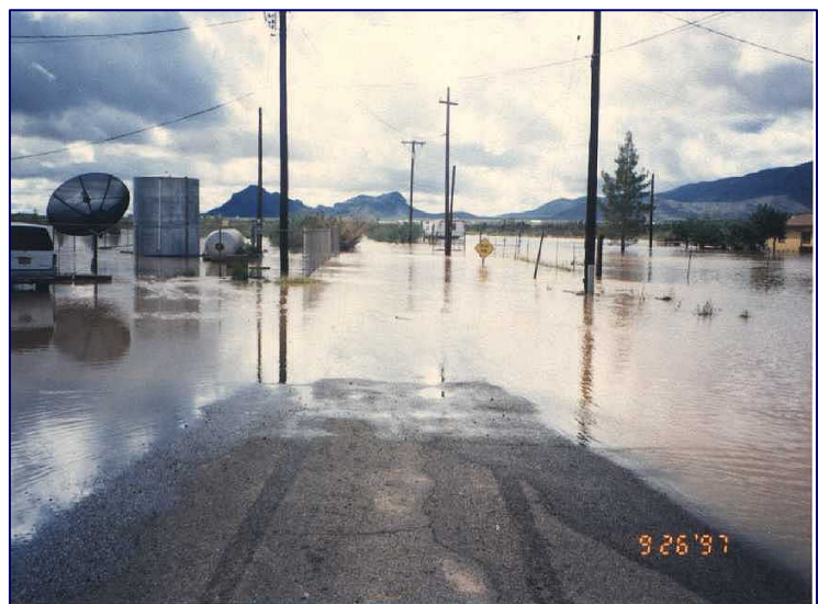
Tropical Storm Nora. September 26, 1997. Flooding, Eagle Eye Road (Rd) and US 60.
