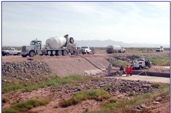
District O & M crews working on structure
