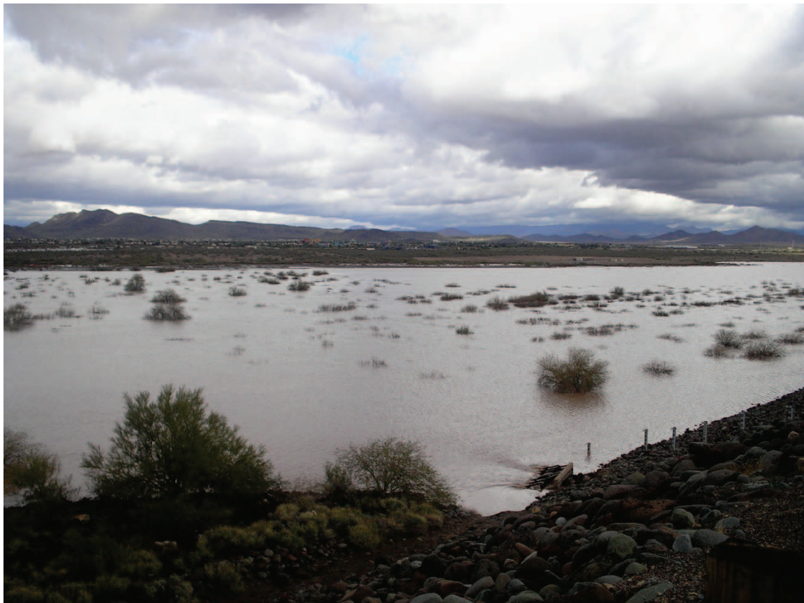
Adobe Dam Pool, ID# 5539 (photo taken January 22, 2010)
