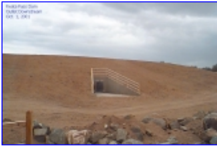
Reata Pass Dam, #4938
