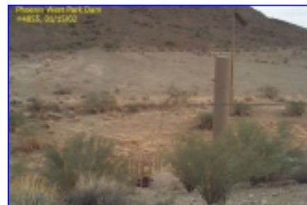
Phoenix West Park Dam, #4858
