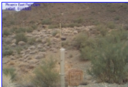
Phoenix East Park Dam, #4848
