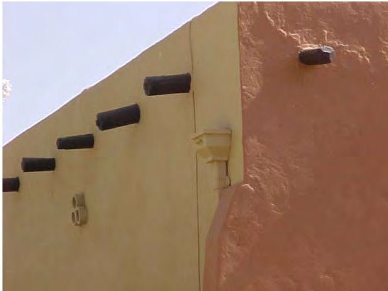
Scupper with downspout.
