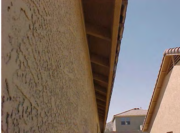
Open soffit with minimal overhang.
