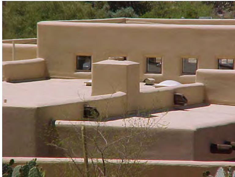
Flat roof with parapet, complex design.
