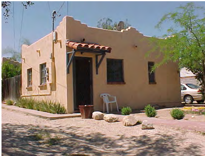
Flat roof with parapet, simple design.
