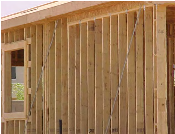
2 X 6 construction and enclosed soffit.
