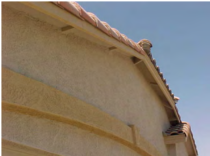
Open soffit with minimal overhang.
