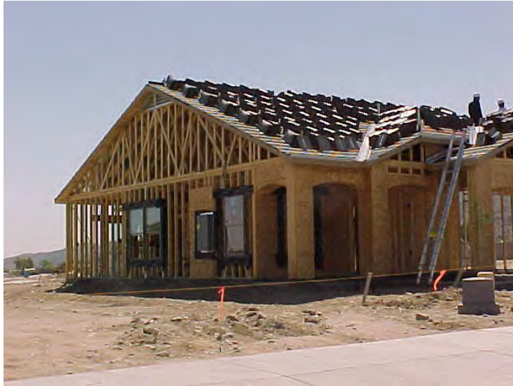
2 X 4 construction with 8 foot wall height.
