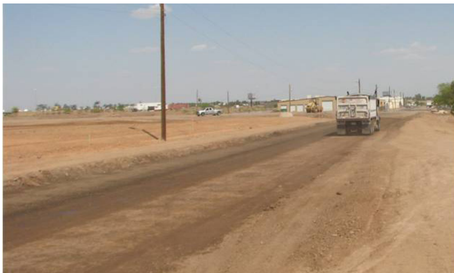
Unpaved Haul Road
