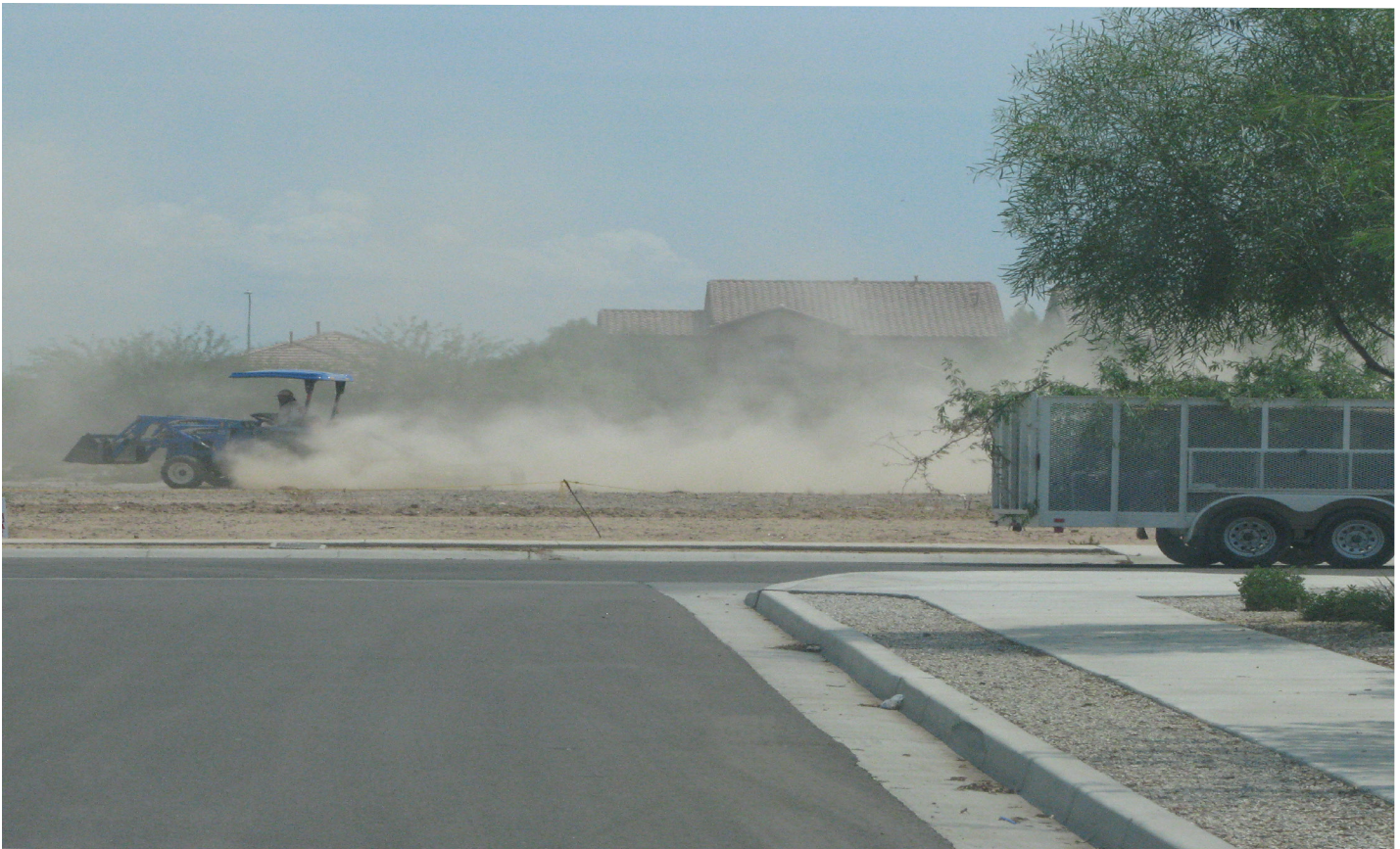
Uncontrolled Dust Emissions During Weed Abatement
