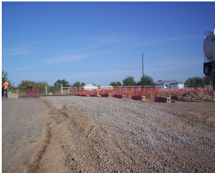
Gravel pad at permitted area entrance/exit
