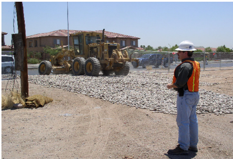
Gravel pad installation at exit
