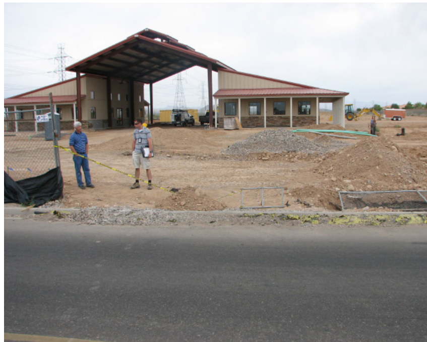
An inspection underway
