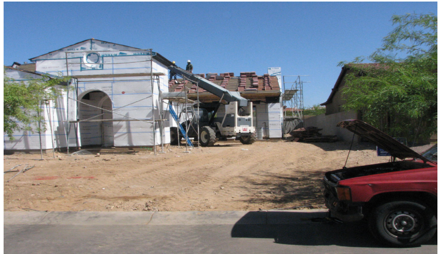
Even a driveway can be an access road
