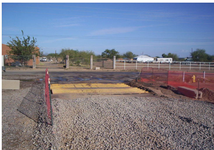
Here a grizzly has been added to the gravel pad as an extra control measure
