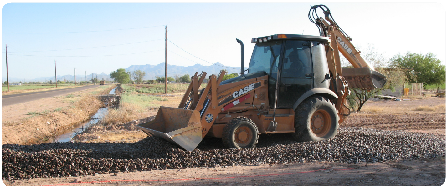
Installing a Gravel Pad
