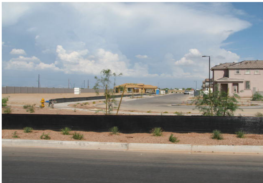
Project nearing completion
