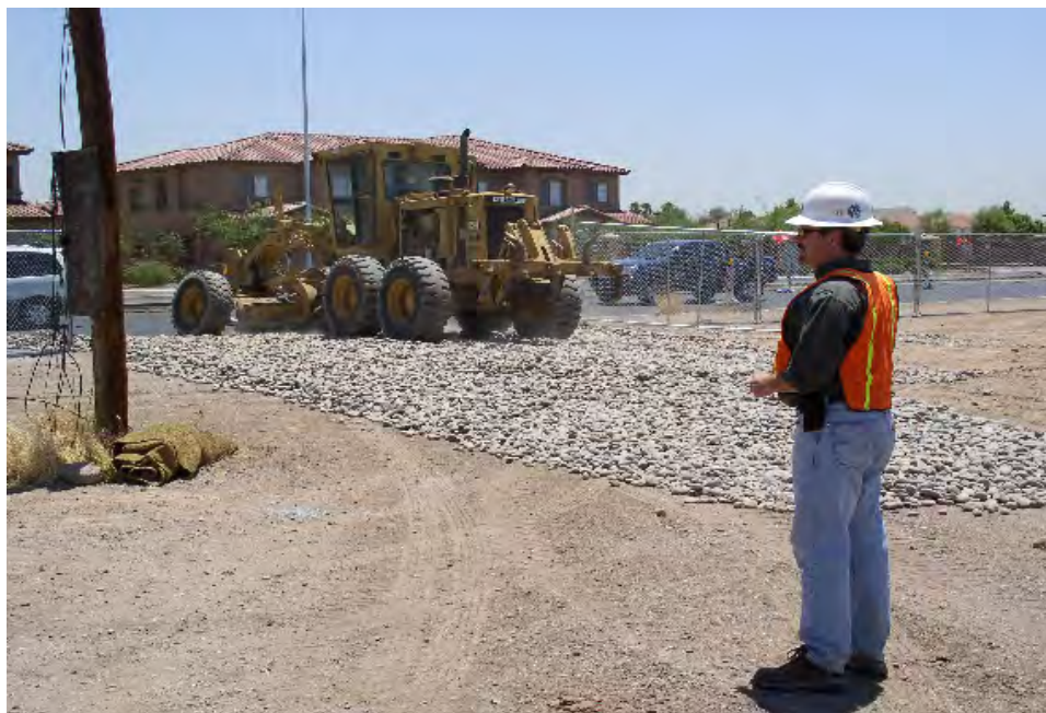
Gravel pad installation at exit
