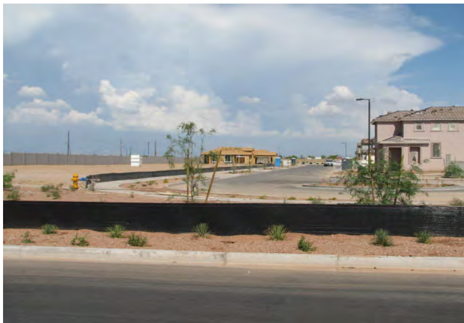
Project nearing completion
