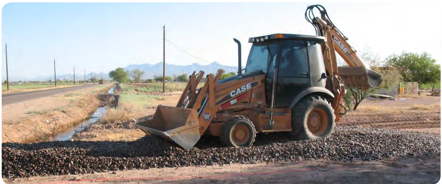
Installing a Gravel Pad
