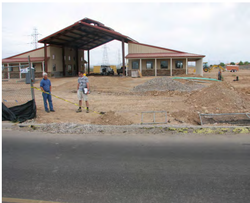
An inspection underway
