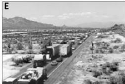
LOS E: Flow becomes irregular, and speed varies rapidly but rarely reaches the posted limit. This represents a marginal service state, where some roadway congestion is inevitable, and is consistent with a road at or approaching its designed capacity.
