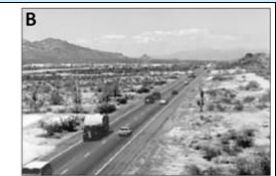
LOS B: Traffic is slightly more congested, with some constraints on maneuverability. Two motorists might be forced to drive side-by-side, limiting lane changes; however, traffic speeds are not reduced.
