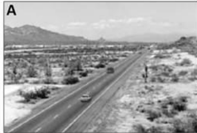
LOS A: Traffic flows at or above the posted speed limit, and all motorists have complete mobility between lanes. LOS A occurs late at night in urban areas and frequently in rural areas.
