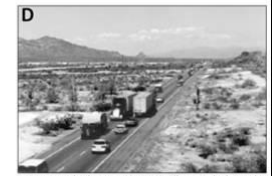
LOS D: Vehicle speeds typically are below the posted speed limit, and motorists' ability to change lanes is reduced due to congestion.
