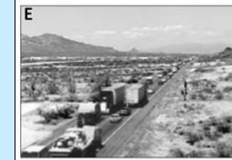
LOS E: Flow becomes irregular, and speed varies rapidly but rarely reaches the posted limit. This represents a marginal service state, where some roadway congestion is inevitable, and is consistent with a road at or approaching its designed capacity.
