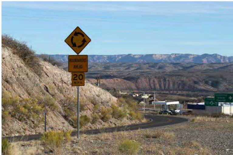
View of advance warning sign for roundabout on SR 89A
