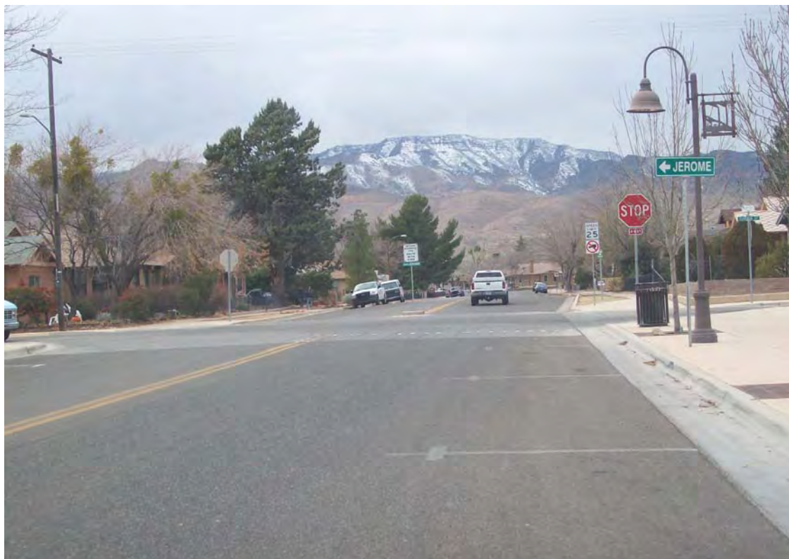
View of ADA compliant crosswalk at 11th St. and Main St.
