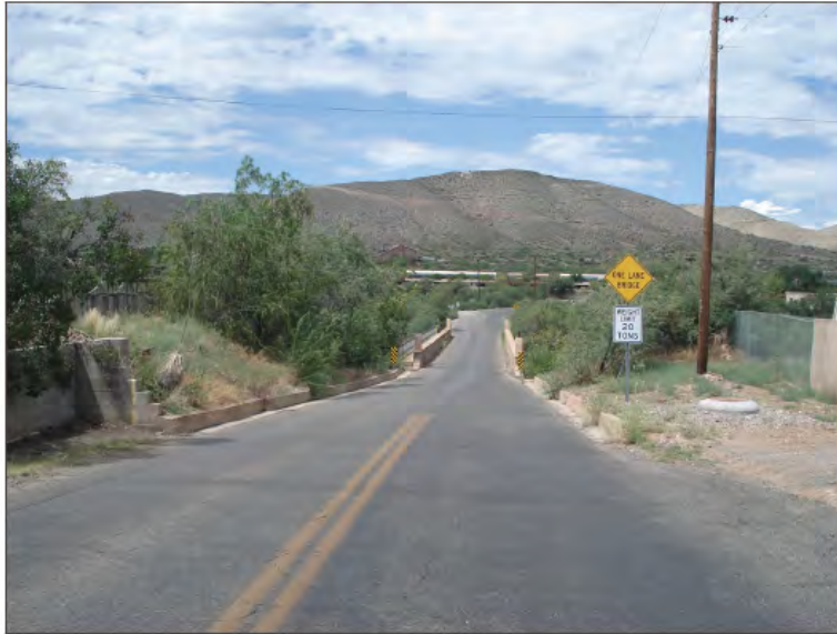
Bitter Creek Bridge, looking north
