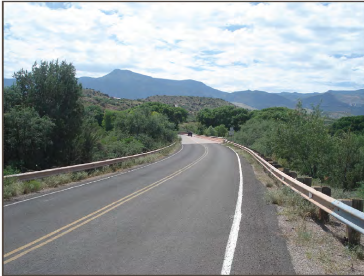
Tuzigoot National Monument Bridge, looking westbound
