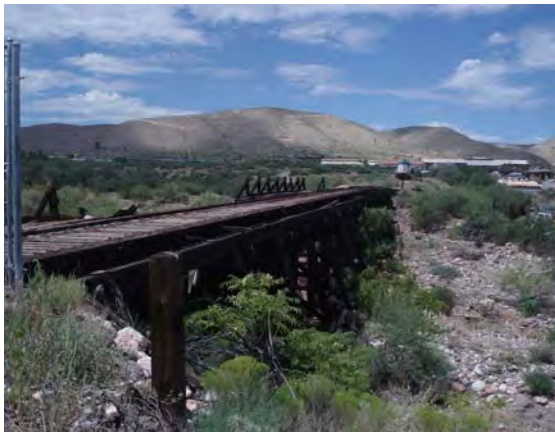
Former rail bridge to be redesigned as a trail
