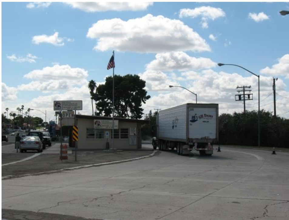
Figure C.28 Yuma (B-8) Port of Entry Facility
