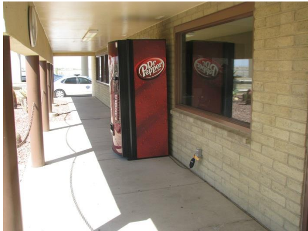
Patio of Administration Building
