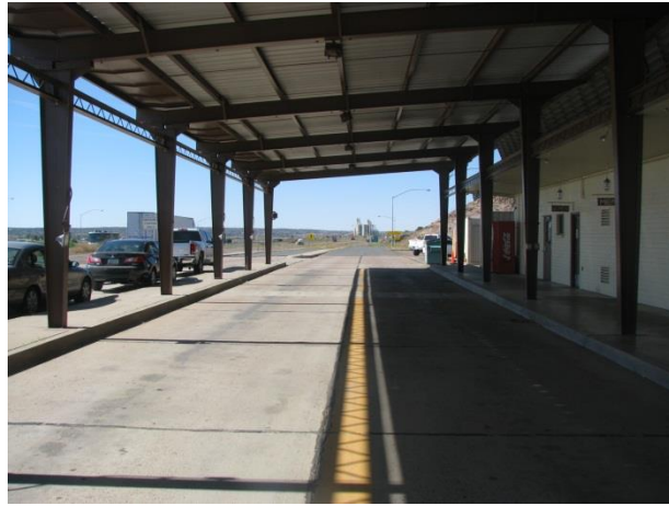
Canopy Structure Attached to Admin Building
