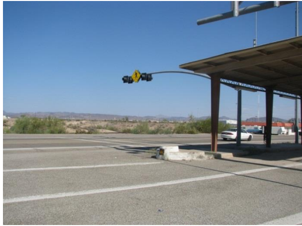
Pedestrian Warning Signage and Beacons
