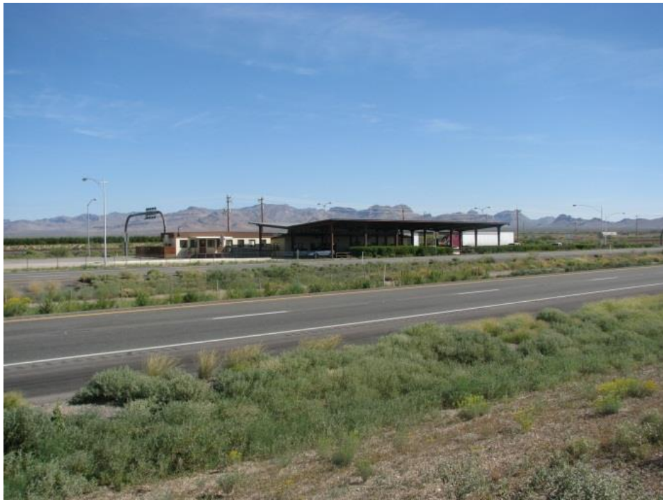
Figure C.13 San Simon Port of Entry Facility
