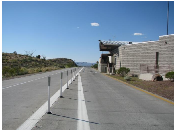
Credential Check/Scale Lane and Bypass Lane
