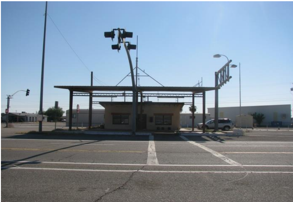
Figure C.37 Parker Port of Entry Facility
