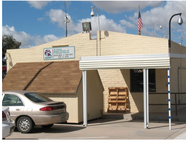
I-8 EB POE Administration Building
