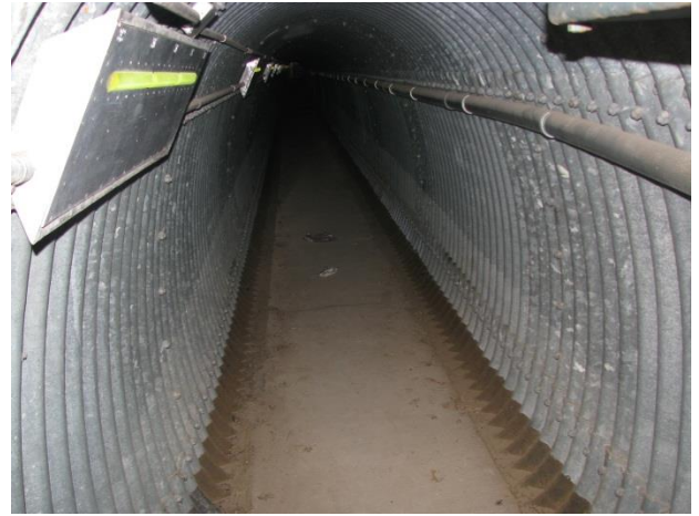
Pedestrian Tunnel Connecting EB/WB POEs
