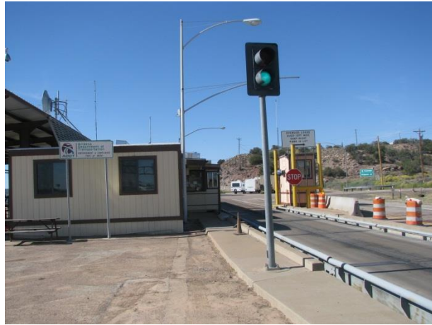
Inbound Static Scale Lane and Admin Building
