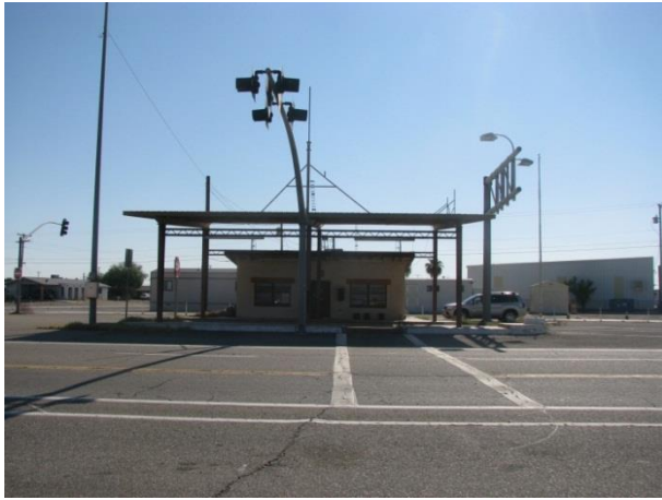
Inspection Canopy and Crosswalk
