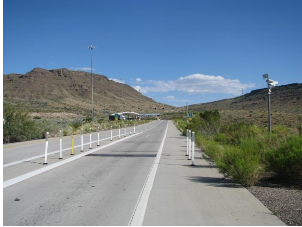
SSWIM Scale on Inbound Off-ramp
