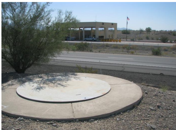
Outbound Pedestrian Tunnel Entrance
