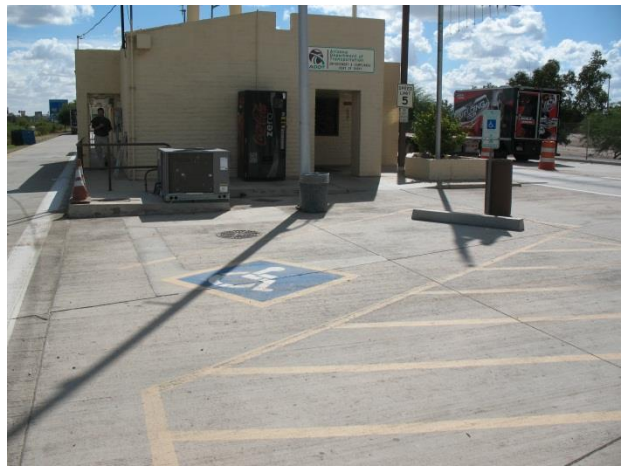
I-8 EB POE ADA-accessible Parking Space
