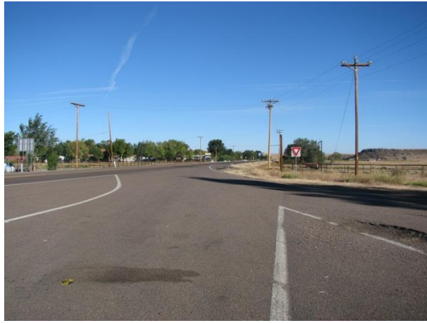
POE On-ramp to US 60
