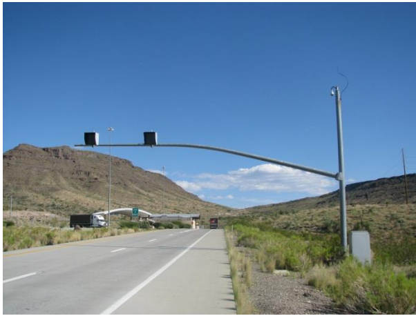
Inbound Lane Control Signal
