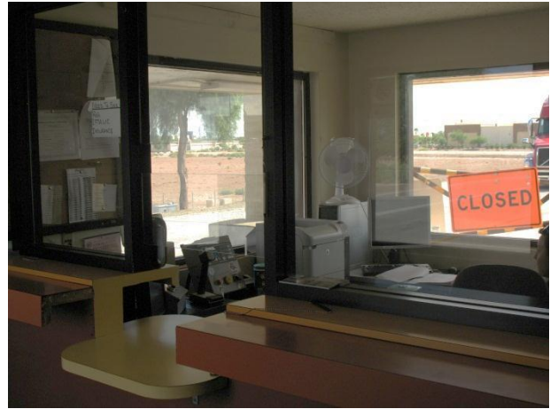
I-8 WB POE Admin Building Interior
