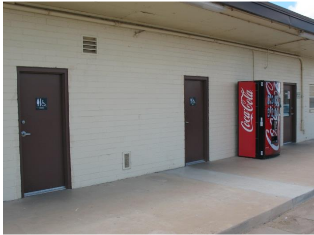
Outdoor Employee Restrooms
