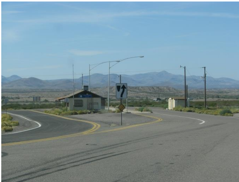
Figure C.31 Duncan Port of Entry Facility
