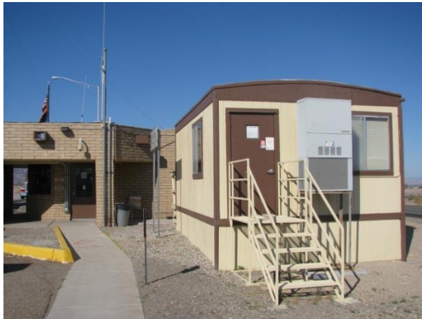
Office Trailer Next to Admin Building
