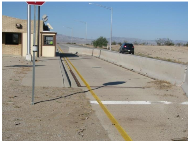
Outbound Static Scale and Concrete Barriers
