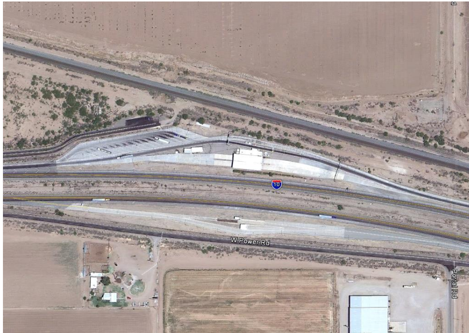
Figure C.14 San Simon Port of Entry Satellite View
