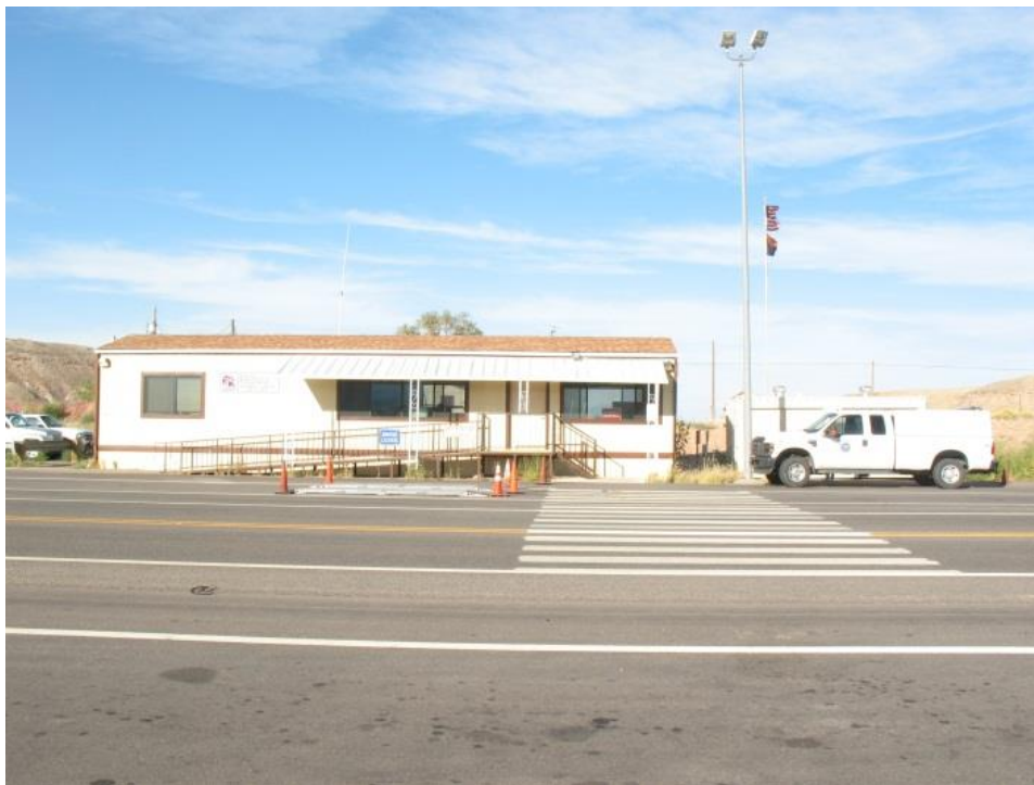
Figure C.25 Teec Nos Pos Port of Entry Facility
