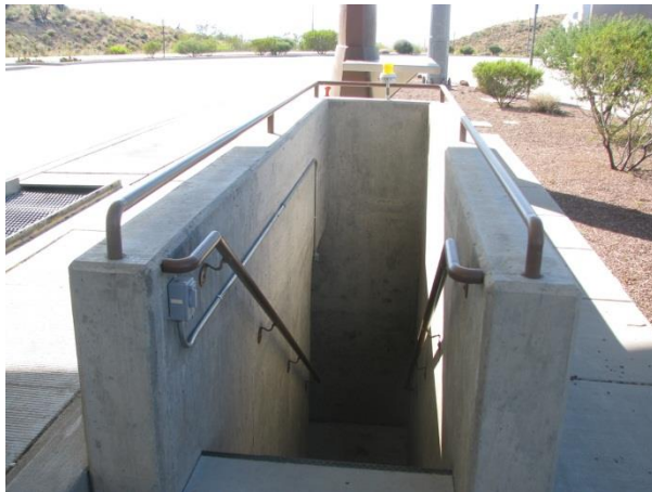
Entrance to Inspection Pit
