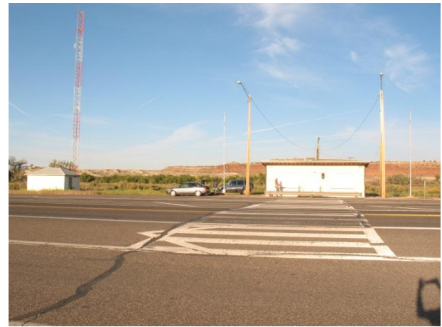
Crosswalk from NB Permit Parking Lane
