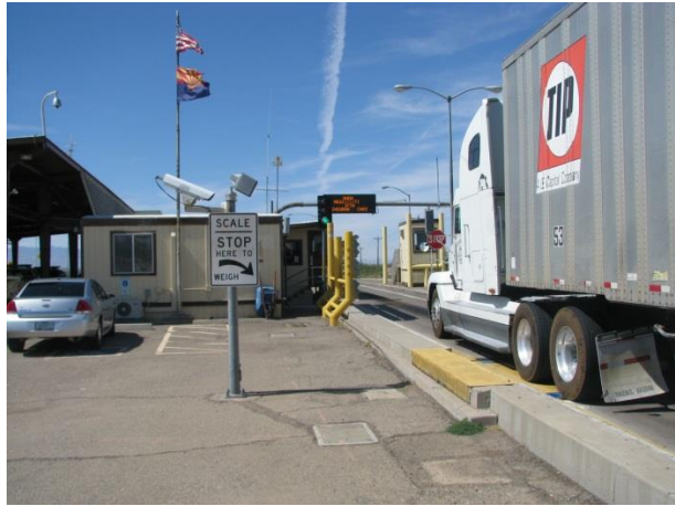
Static Scale with LCS and Overhead CMS
