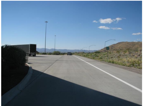
Return Loop and Truck Parking Lot
