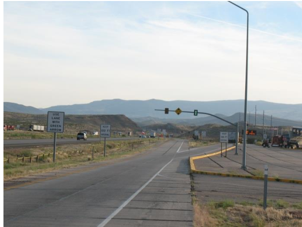
Lane Control Signal on Inbound Off-ramp
