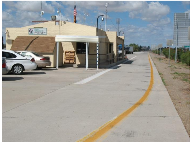
I-8 EB POE Bypass Lane East of Building
