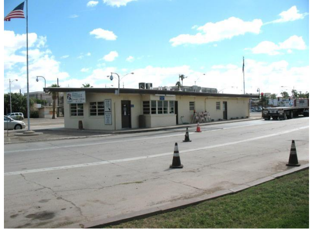
Inbound Lanes at Admin Building
