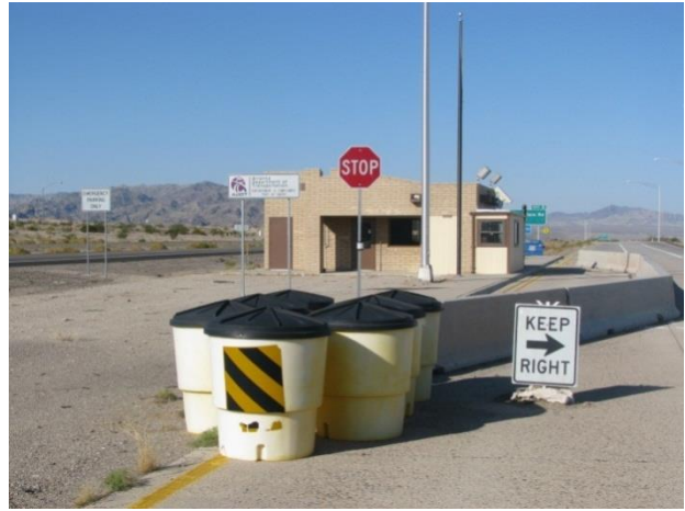
Outbound POE Admin Building
