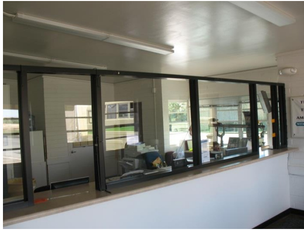
Customer Service Windows
