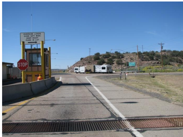
Inbound Oversize Truck Lane and Booth
