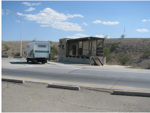
Storage Building and Truck Parking
