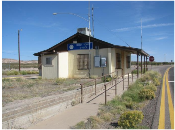
Pedestrian Ramp Outside Admin Building
