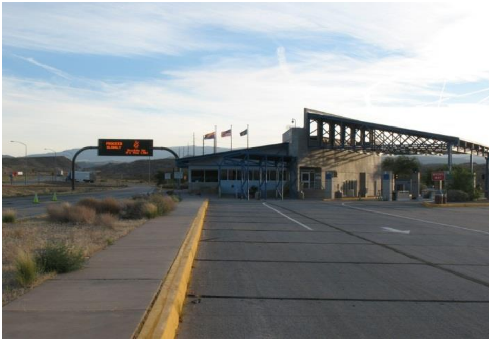
Figure C.7 St. George Port of Entry Facility
