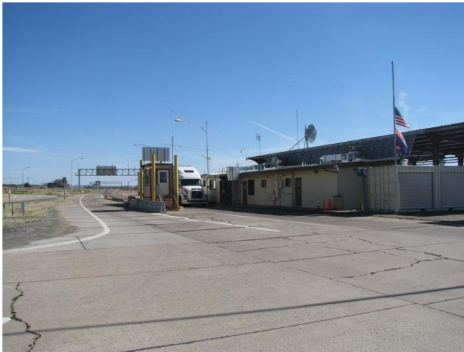
Figure C.10 Sanders Port of Entry Facility
