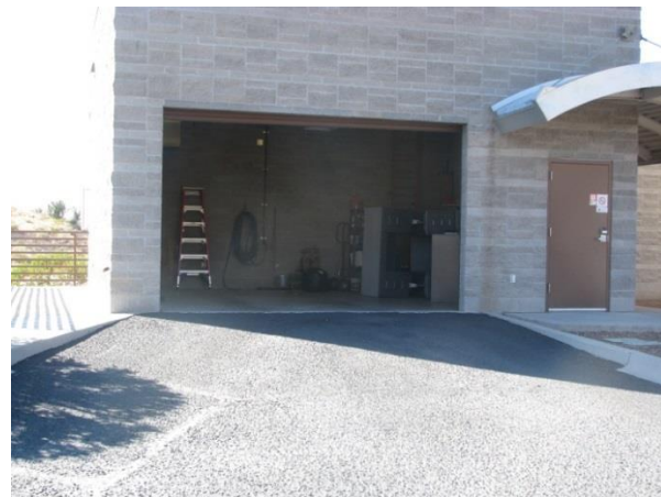
Garage and Storage Room
