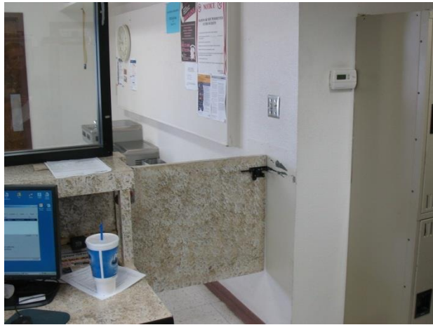
I-8 EB Admin Building Unsecure Swing Gate
