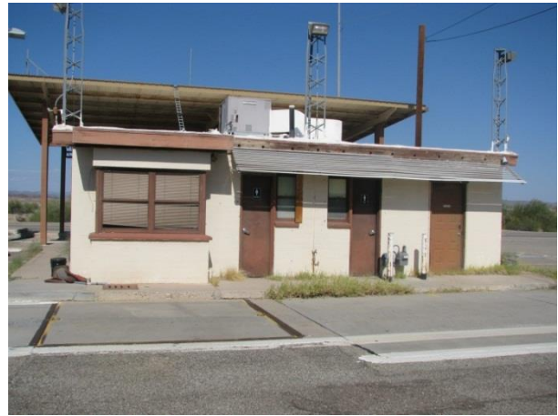
Admin Building and Static Scale
