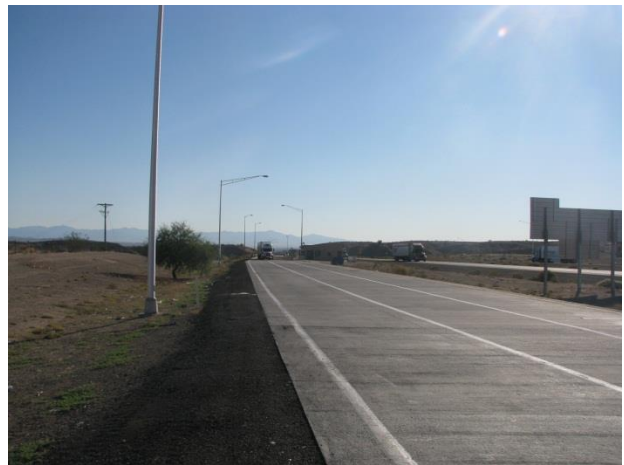
Outbound Credential Lane and Bypass Lane
