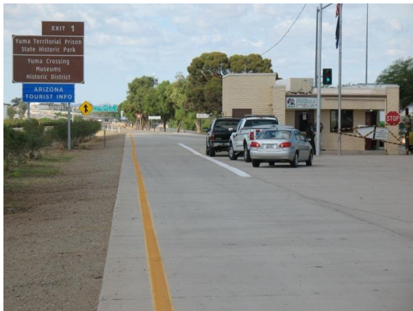
I-8 WB POE Bypass Lane West of Building
