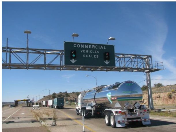
Overhead LCS on Inbound Off-ramp
