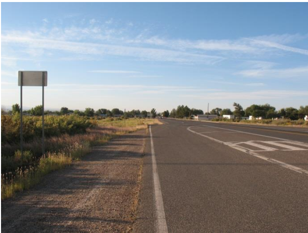
NB Permit Parking Lane
