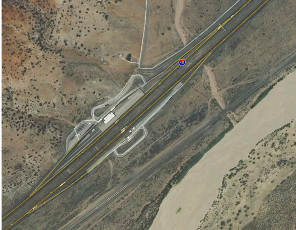
Figure C.11 Sanders Port of Entry Satellite View
