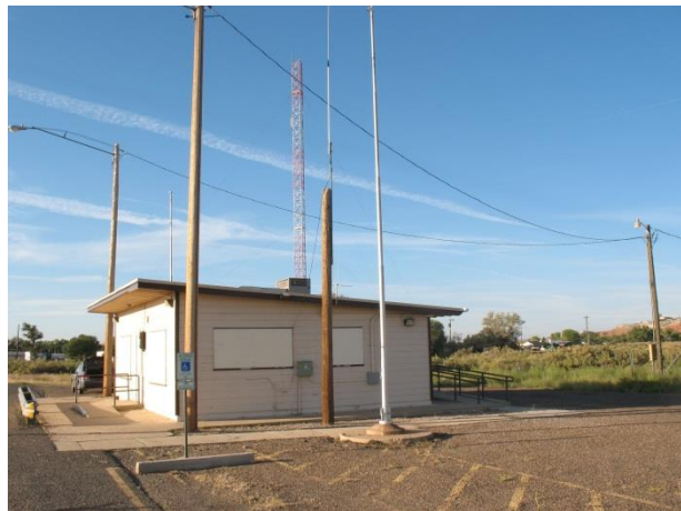
ADA-accessible Parking Space and Ramps
