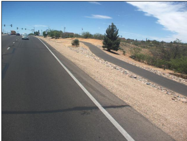
Existing Shared Use Path on SR 92 at MP 321.2 (Sierra Vista)
