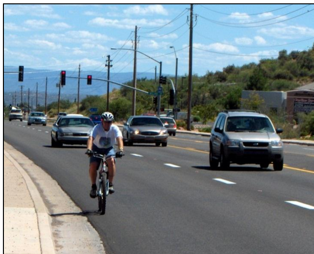
Wide curb lane on SR 89A
