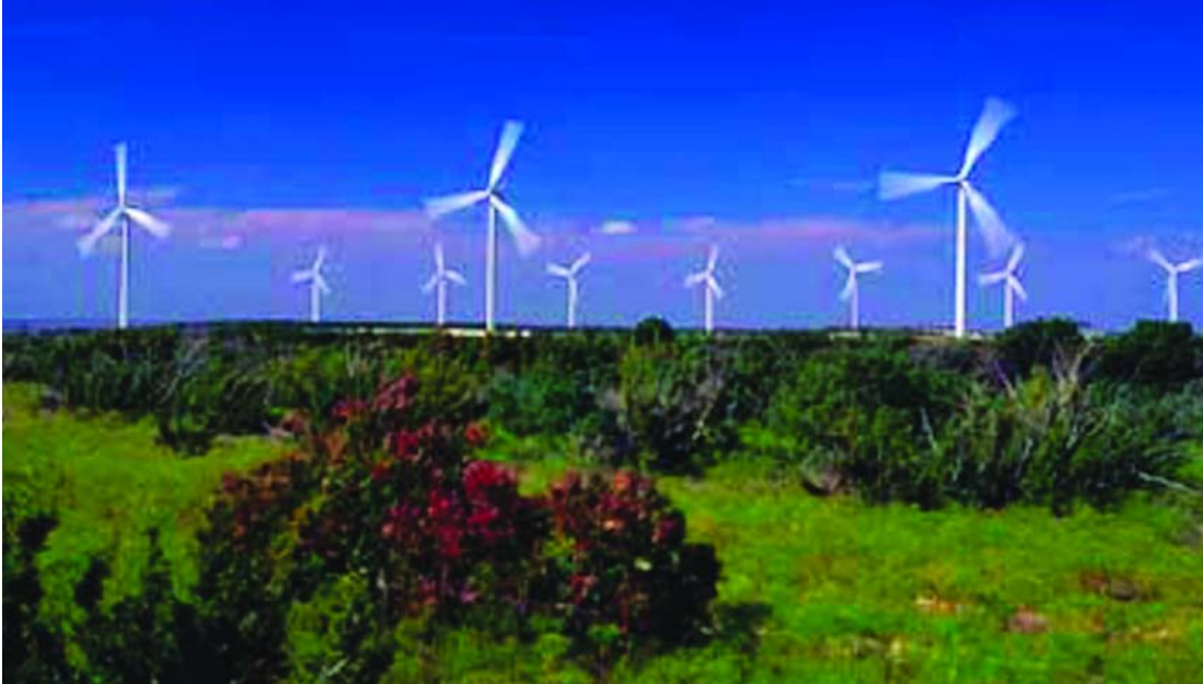
Trent Mesa Wind Project in west Texas.
