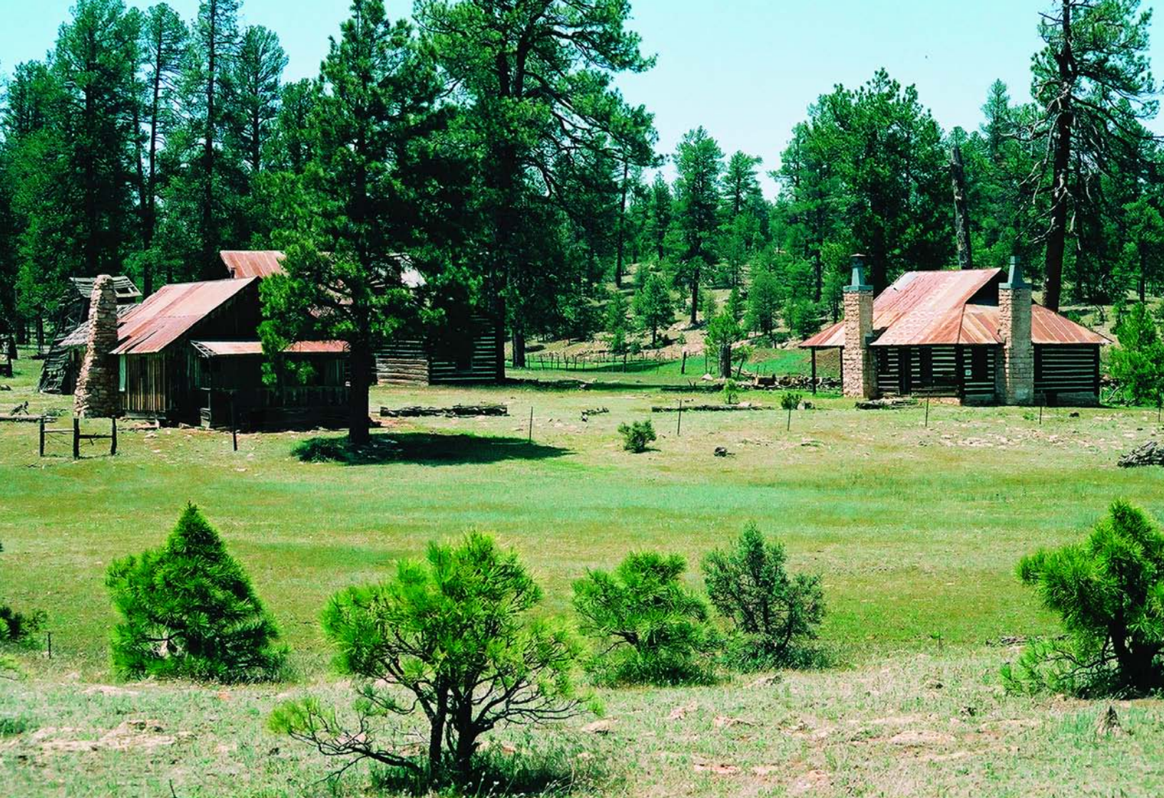
Moqui Ranch (above) and other ranch-owned properties throughout the national forest may present some opportunities for limited home site development.
