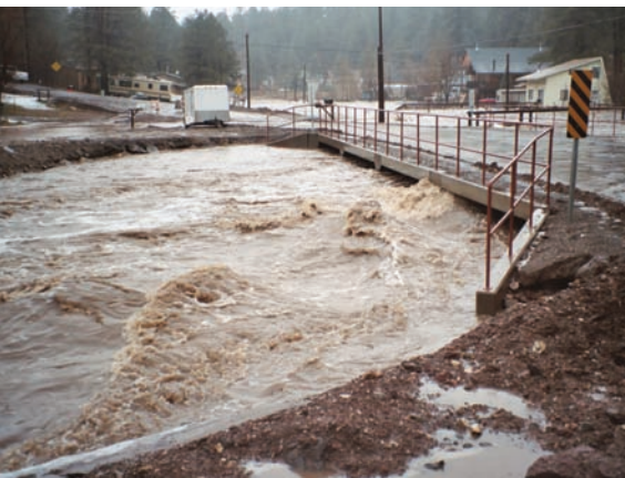
Infrequent but severe flooding can occur along Pumphouse Wash.
