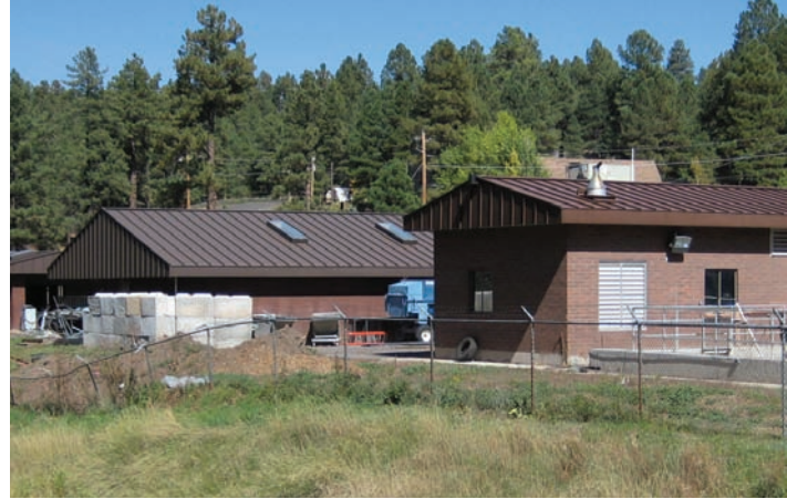
KVID wastewater treatment plant.
