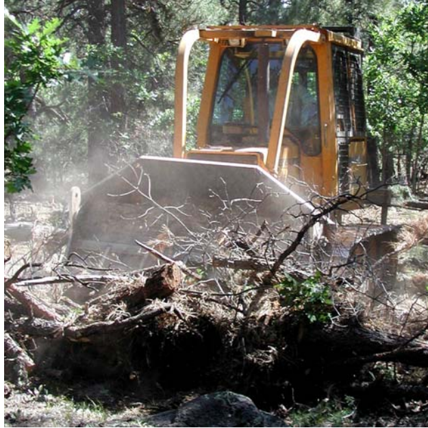
Dozer piling. Source: Kaibab National Forest
