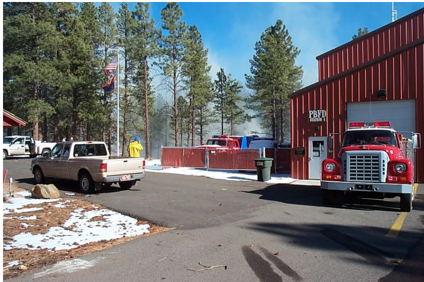
Parks-Belmont Fire Station, pile burning. Source: Kaibab National Forest
