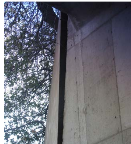
Spring Canyon Structure
