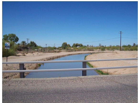
The East Main Canal bisects the residential area in the East Reservation
