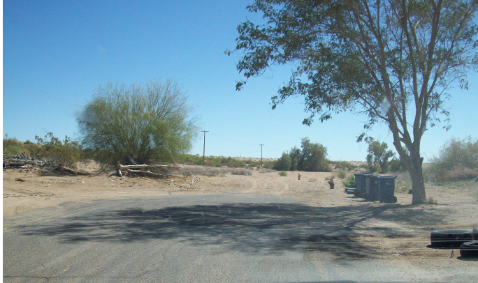
Cul-de-sac at the end of Cottonwood Lane. This cul-de-sac needs to be widened to accommodate emergency vehicles and signed and marked appropriately
