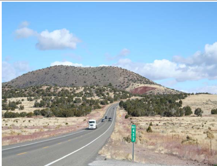
Leupp Road, at MP 433
