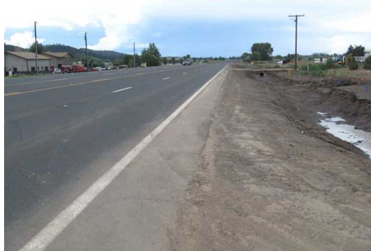
US 89 at Copeland Road
