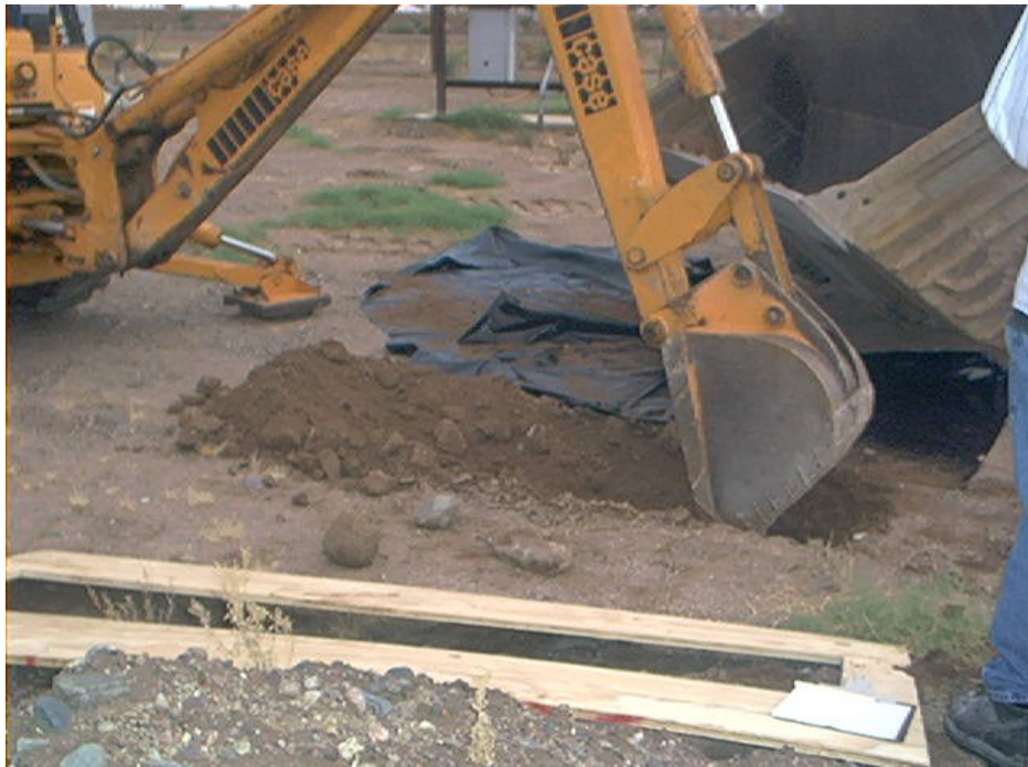
Figure 47: Hole is Excavated Using the Backhoe.
