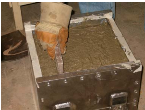
(e) Leveling Concrete
