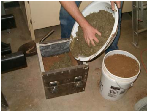
(c) Concrete Poured into the Box
