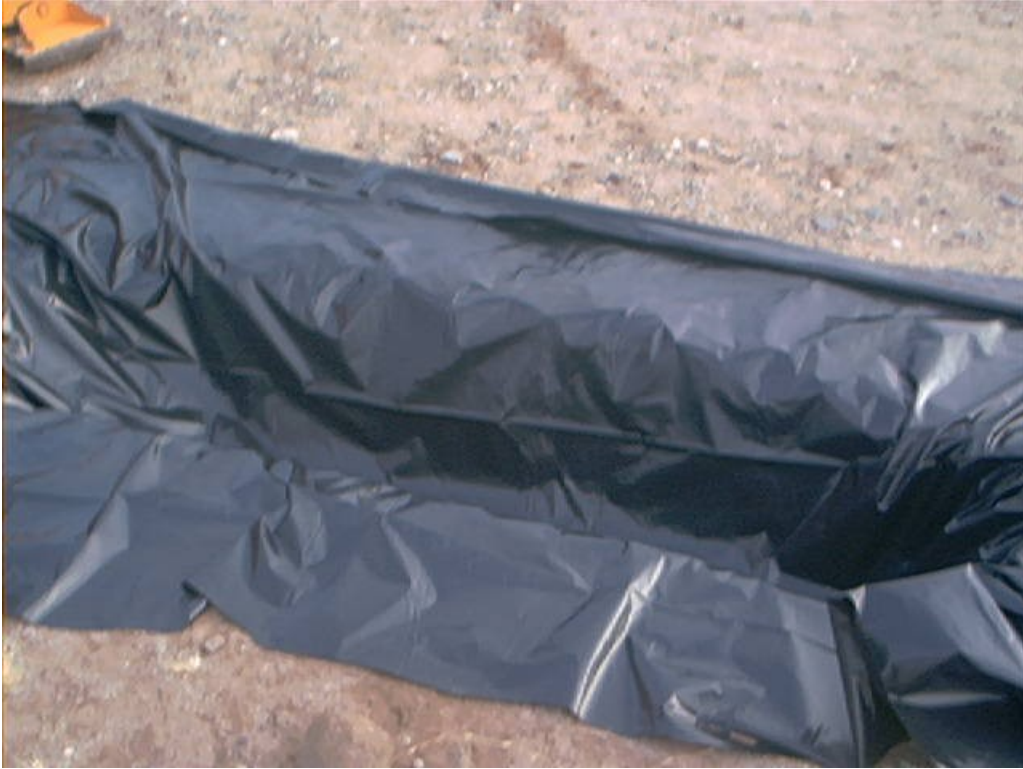
Figure 49: The hole is lined with a Plastic Sheet.
