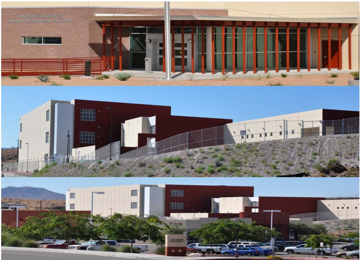
Mohave County Capital Improvement Project—Adult Detention Facility, completed 2010
