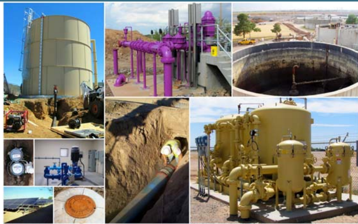
Example projects include storage tanks, meters, wells and booster pumps, arsenic treatment systems, distribution line rehab, well drilling, solar, sewer rehabilitation, wastewater plant upgrades, and upgrades for reclaimed water, sewer rehab and replacement.
