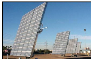
PTL Solar Panels
