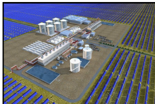
Solana APS Plant
