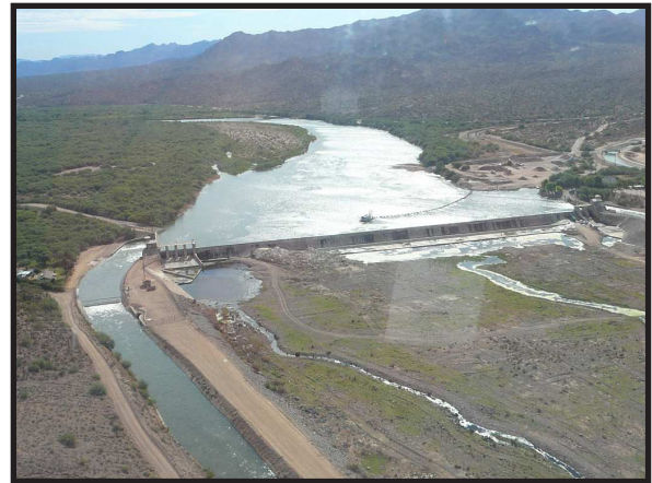
AMA Planning Area, Granite Reef Diversion Dam. The Salt River is ephemeral below Granite Reef Diversion Dam.
