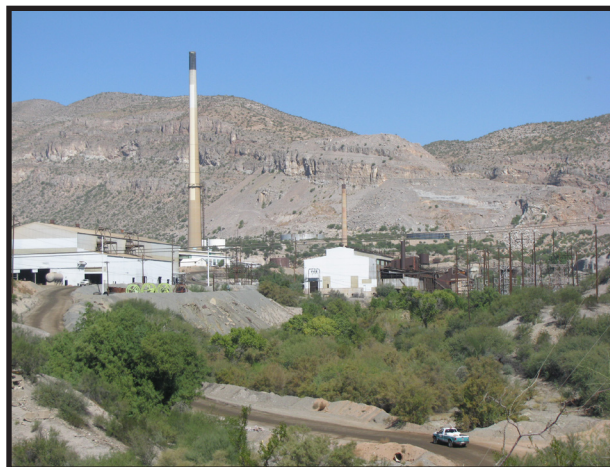
ASARCO Hayden Smelter, Lower San Pedro Basin. All of the industrial demand, the largest demand sector in the Lower San Pedro Basin (almost 16,000 AFA), is met by groundwater, which is also the primary water supply for agricultural and municipal purposes
