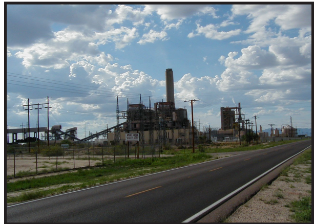
APECO Power Plant, Willcox Basin. Almost all the water supply for this basin is found in basin fill deposits.
