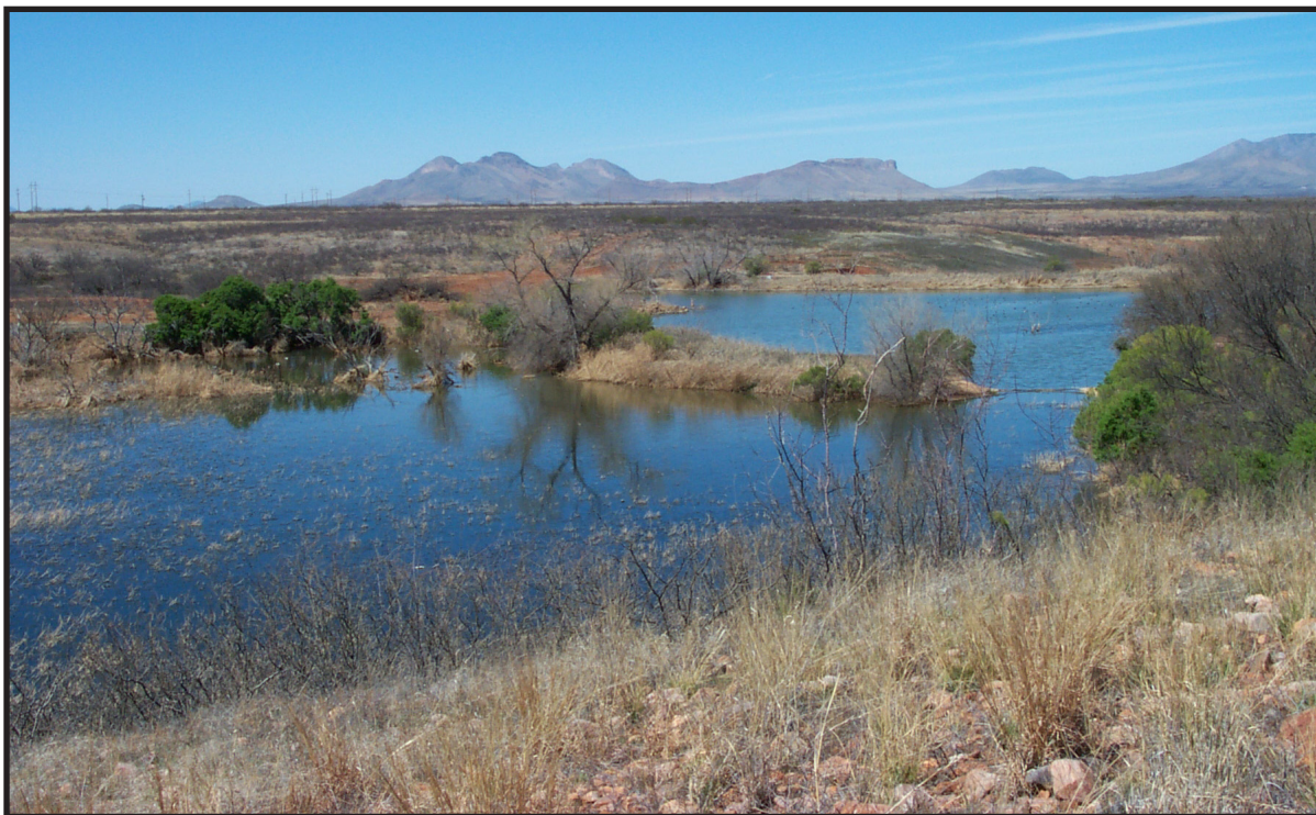
Recharge basins at Fort Huachuca, Upper San Pedro Basin. Approximately 2,380 acre-feet of effluent were recharged to the aquifer at the Fort Huachuca and Sierra Vista Recharge facilities in 2007.
