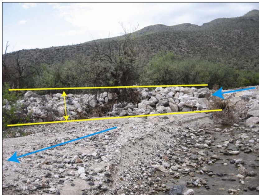
Figure 8. 2006 debris-flow deposits in Soldier Wash upstream of the Mount Lemmon Short Road. Yellow lines highlight boulder snout deposited after, and on top of, an earlier pulse that likely plugged the bridge. Blue arrows show direction of flow. Photo: P.G. Griffiths, Sept. 12, 2006 (see Solder Canyon discussion below).
