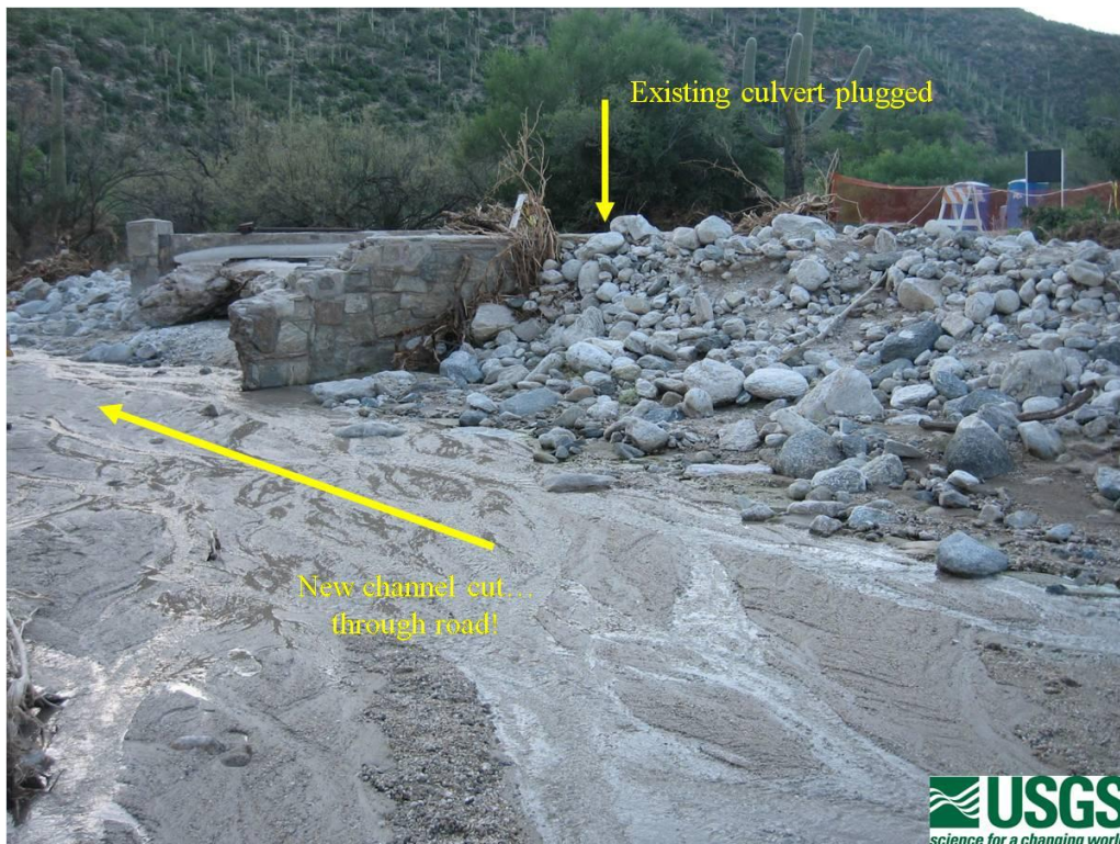
Figure 3. View downstream of the remaining part of Rattlesnake bridge. Photos: US Geological Survey.
