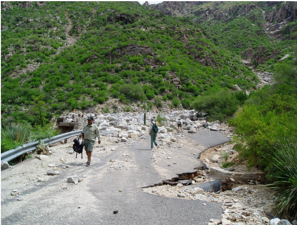
Figure 12. Tram Stop 9. Debris flow chute in upper right of photo.
