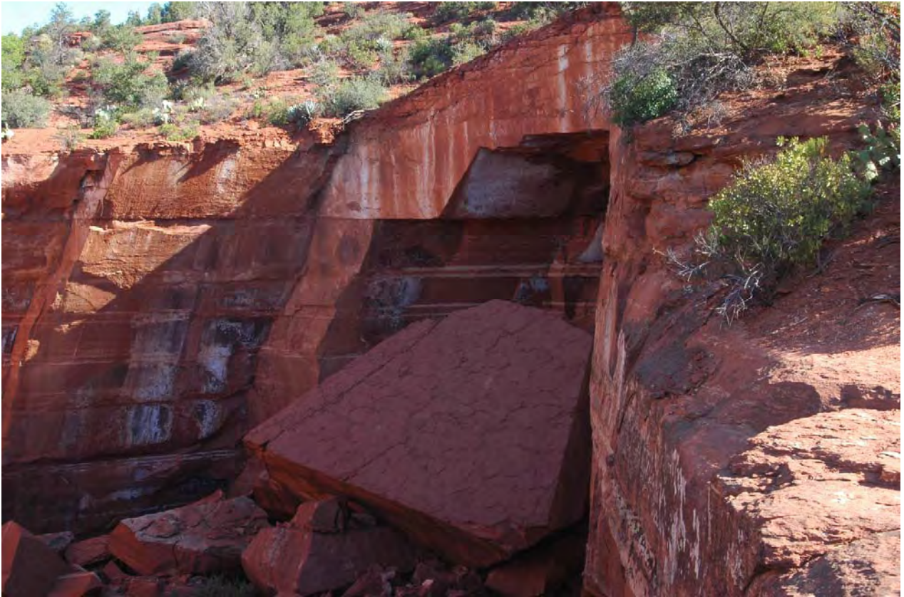
Figure 6. Devils Kitchen sinkhole after 1995 rock fall. This 2009 photograph shows the large sandstone block at the north end of the sinkhole that rotated forward during the 1989 collapse. Another piece of the northern joint face just above it fell off the cliff in 1995 and landed behind the big slab (compare with fig. 5). In the twenty year interval since the 1989 collapse, weakly acidic rainwater has dissolved most of the thin white coating of caliche ( \text{CaCO}_3 ) on the near vertical joint face. Geologic plan map (fig. 13) and cross sections (fig. 14) show the rock fall locations. Note the bell-shaped, downward enlarging rock fractures in the northwestern corner of the sinkhole. Arcuate fractures such as this are localized around sinkhole sites and have been superimposed upon the arrow-straight and nearly vertical northwest-trending rock joints.
