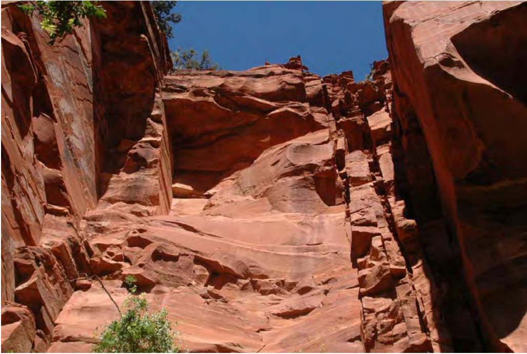
Figure 32. Northwest-trending joints on west wall of Red Canyon sinkhole. Drain is 98 feet (30 m) directly below these fractures.
