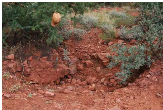
Figure 36. Photograph of 4543 sinkhole. Despite its small size, Air pressure changes allow air to exit or enter, indicating the presence of a large cavity below ground level.
