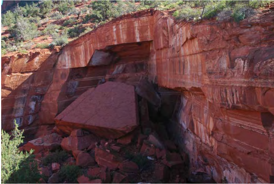
Figure 16. Devils Kitchen sinkhole in September 2008. Note the fresh, angular rock breaks and vestige of white caliche that marks the pre-1989 boundary of the sinkhole.
