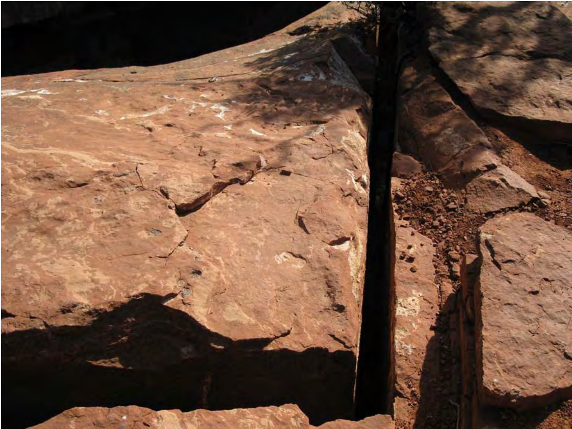
Figure 15. Open fracture in west edge of Devils Kitchen sinkhole. This fracture has been widening over the past several decades. What was once a 2 inch (5 cm) break is now 7-9 inches wide (18-23 cm). Frost heaving and rock wedging will ultimately cause this piece, and another similar block to the north, to break loose and “unload” the southwestern corner of the sinkhole in a future collapse. The entire outcrop to the southwest of this fracture has already been broken with arcuate fractures.
