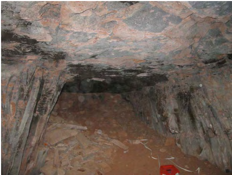
Figure 21. Interior of Mitten Ridge sinkhole. The walls show abundant, closely spaced stress fractures in Schnebly Hill Sandstone that widen downward. Massive sandstone caprock appears to be unbroken, indicating that this is the extreme top of a column of collapse breccia. Note the black soot from prehistoric occupancy on the ceiling.
