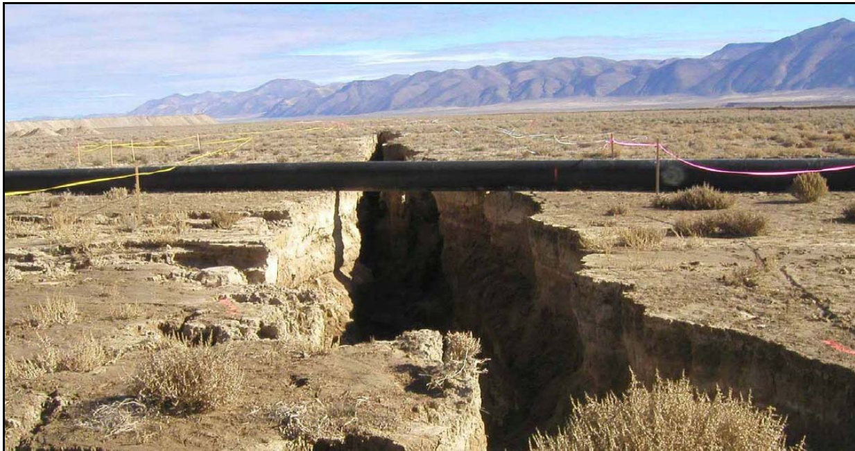
Fig. 9 – Fissure gully crossing below above-grade pipe at a mine facility in Nevada (photo by AMEC presented in 2004 ADOT workshop)
