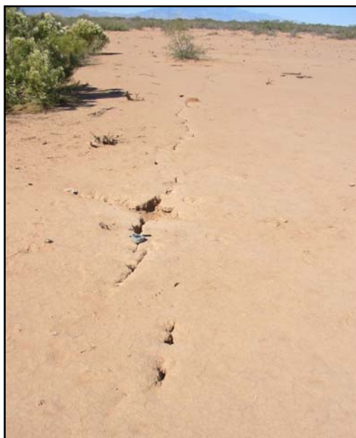
Fig. 3 - Incipient fissure cracking near Bowie, Arizona (photo by Ken Euge)
