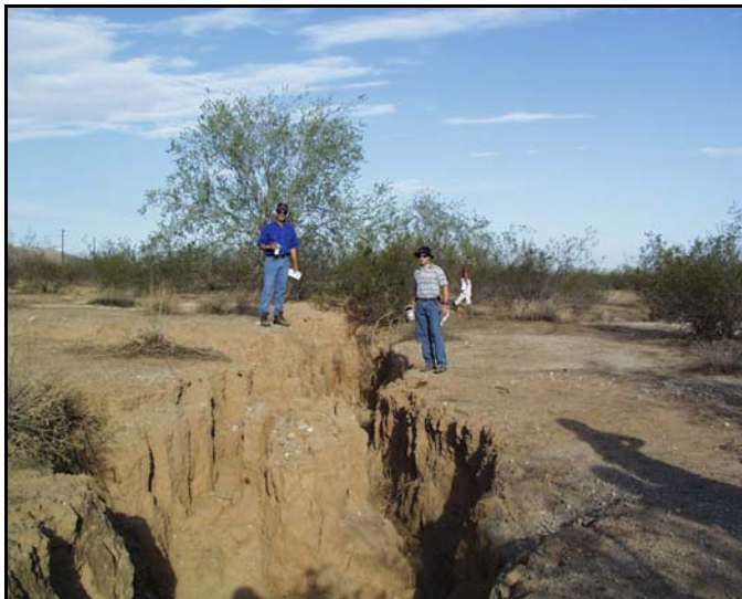
Fig. 1 - Differential displacement along fissure near Hunt Hwy in Pinal County (photo by Ken Euge)
