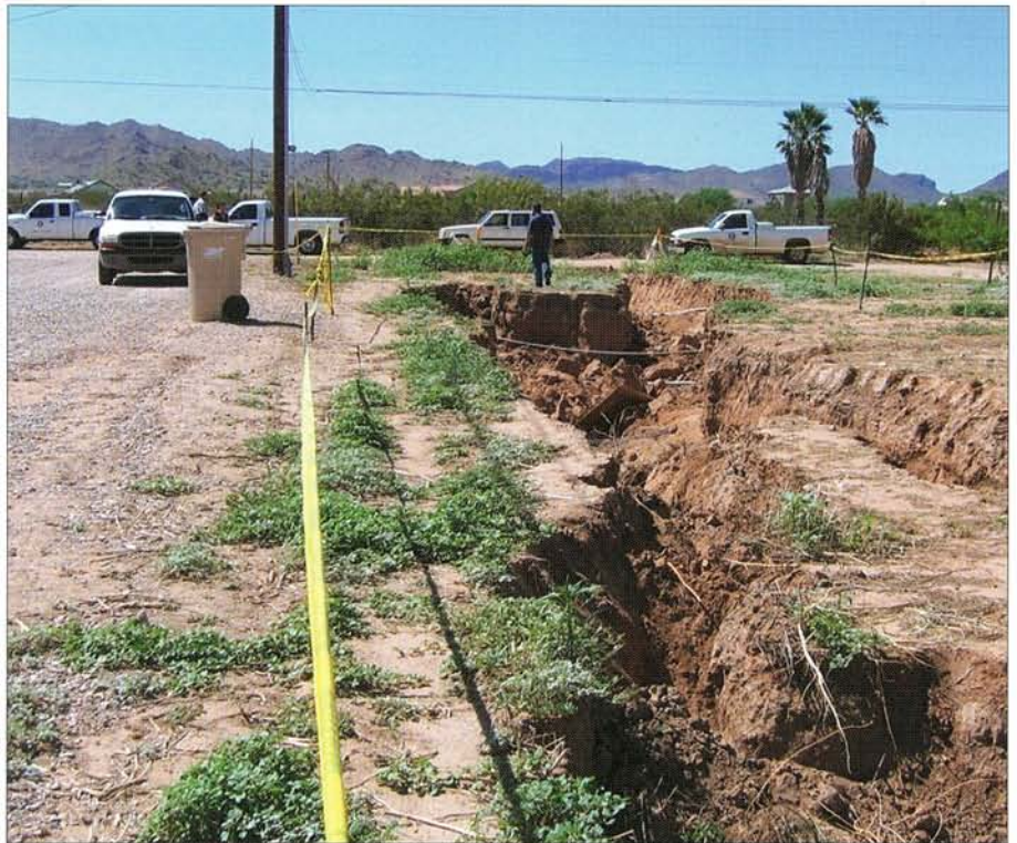
Figure 1: Earth fissure near Chandler Heights, Maricopa County, August 2005. Earth fissures range from insipient, where they are characterized by discontinuous, pock-marked ground and hairline fractures, to mature features miles in length and hundreds of feet deep, with associated gullies at the surface that are more than 10 feet wide and several tens of feet deep. (Photo by Ray Harris)
