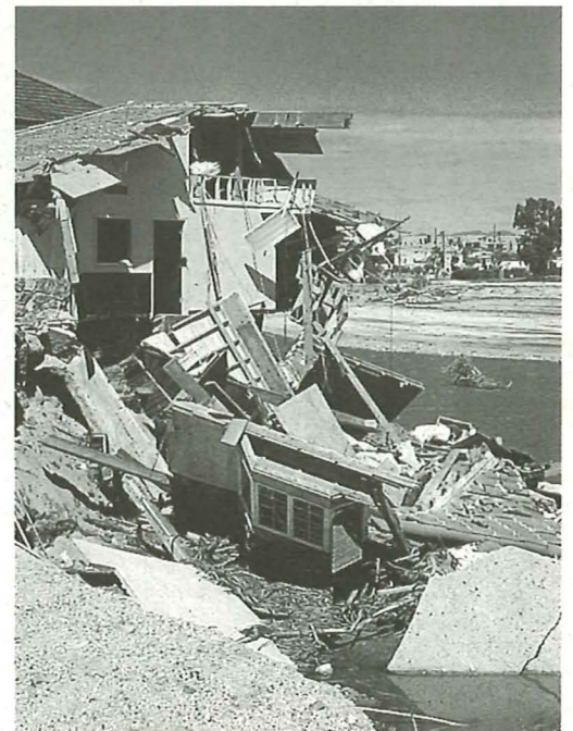
Building destroyed by the October 1983 flood on the Rillito River in Tucson.
