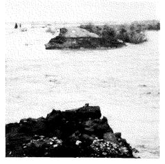
Figure 12. Breach in an artificial levee on the Little Colorado River near Winslow on January 7. The breach was closed on January 14 before another series of storms caused flooding that came within 2 feet of the crest of the repaired levee. Photo by Chuck Williams, Navajo County Flood Control District.
