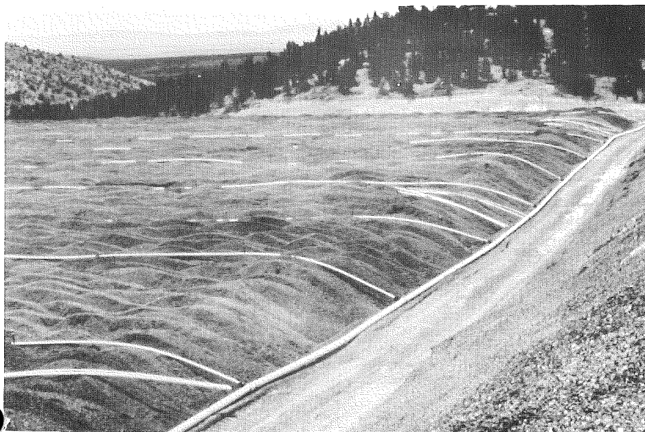
Figure 1. Typical heap-leaching operation for recovery of gold from crushed ore using dilute cyanide solutions. Heap leaching of crushed ore usually involves 30- to 60-day leach cycles and yields gold recoveries of 60 to 90 percent.
