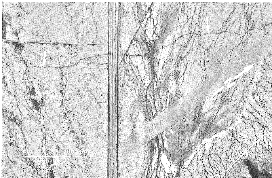
Figure 2. Aerial view of earth fissure crossing Interstate Highway 10 (I-10) between the town of Picacho and Picacho Peak. Photo taken on December 9, 1963 by the Arizona Department of Transportation.
