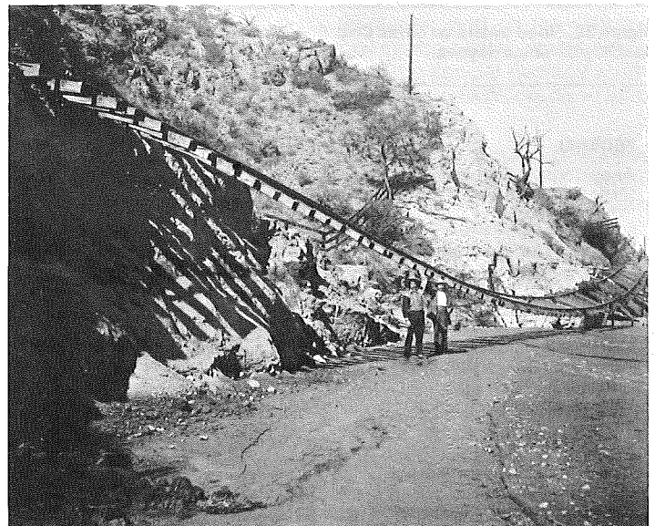
Figure 3C. Bank erosion left the Southern Pacific Railroad track dangling at Tucson, late 1800s. Photo courtesy of University of Arizona Library, Special Collections, Tucson.
