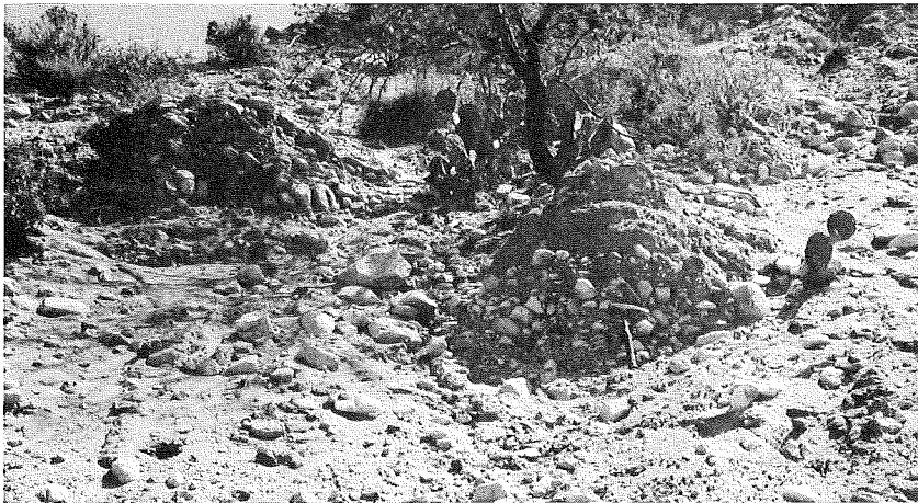
Photo 8. Close-up of photo 7. Looking into failure plane. More resistant flatlying coarse beds remain in place. Failure plane inclined at 35°
