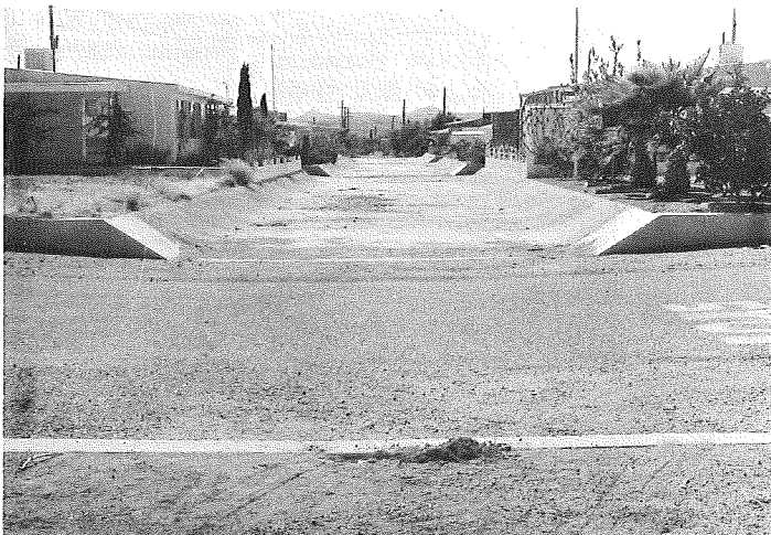
Fig. 4. Stream channel modification such as this one shown above is common to new subdivisions.
