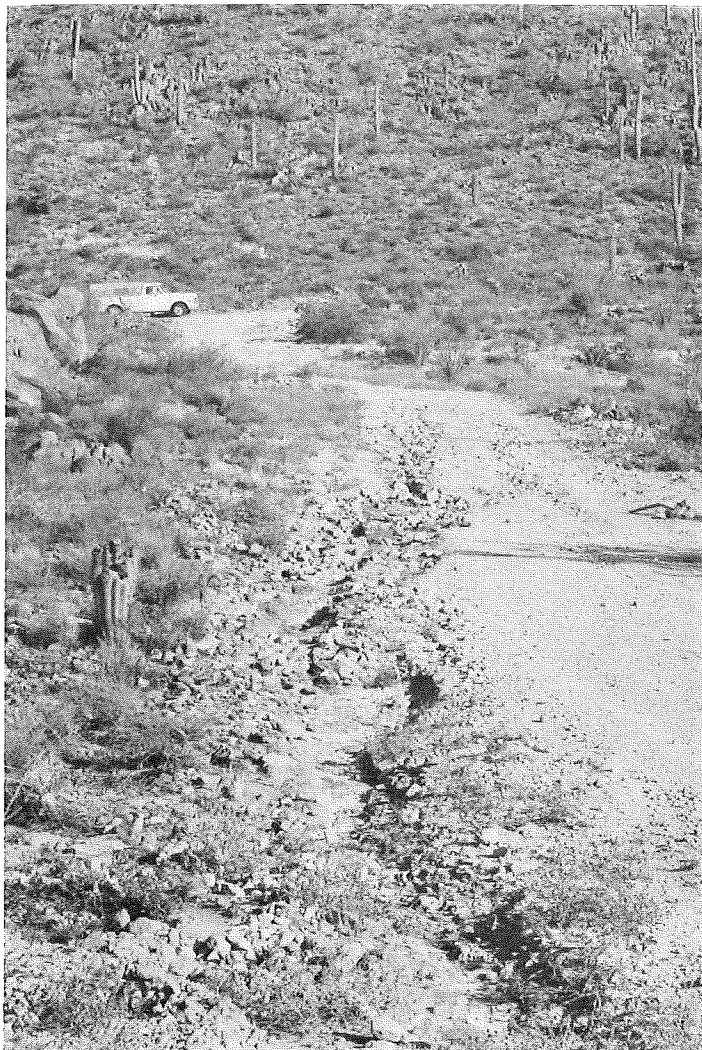
Fig. 3. This gully-cutting form of destructive erosion on a subdivision road was caused by human activity (bulldozer grading?).
