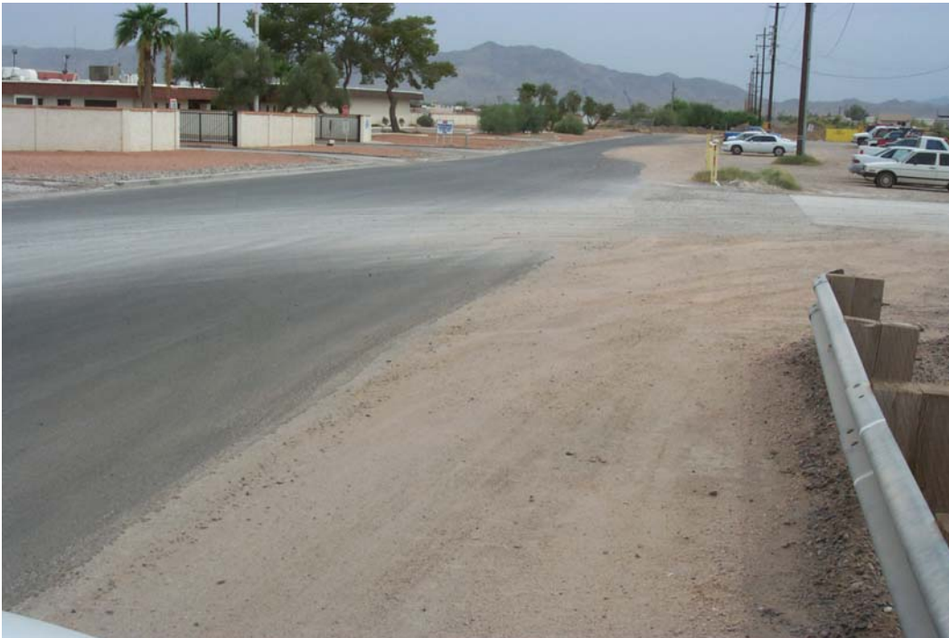
Figure D-2. Sample #2 taken on south bound lane of 43 rd Avenue at Elwood Street, 445 feet north of the origin (area dimensions = 6 feet by 18 feet). Photo is looking southwest.
