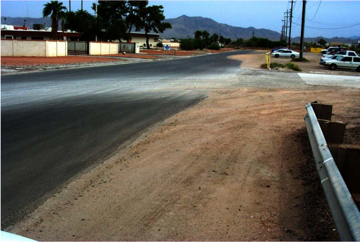
Figure 4-5 – Trackout on 43 rd Avenue, looking south and north respectively.
