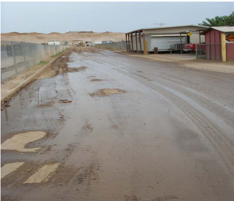
Figure D-6. Example of trackout on exit road onto 43 rd Avenue & Elwood Road, that is used by the Glenn Weinberger Company. Photo is looking east.
