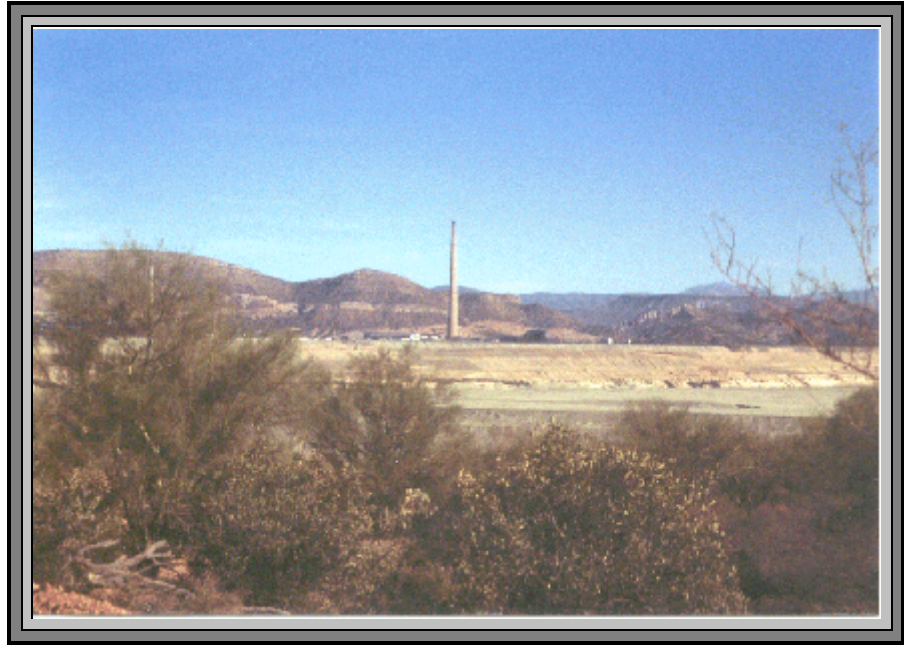
Figure 8. The San Manuel copper mining complex, including the smelter smokestack and tailings piles are shown in this photo. Groundwater from the underground mining operations had been pumped at a rate of 4,000 gpm and applied to the tailings piles for dust control. This practice ended in January 2002 when a four inch cover of rock material capped the more than 3,000 acres of tailings dumps 23 .
