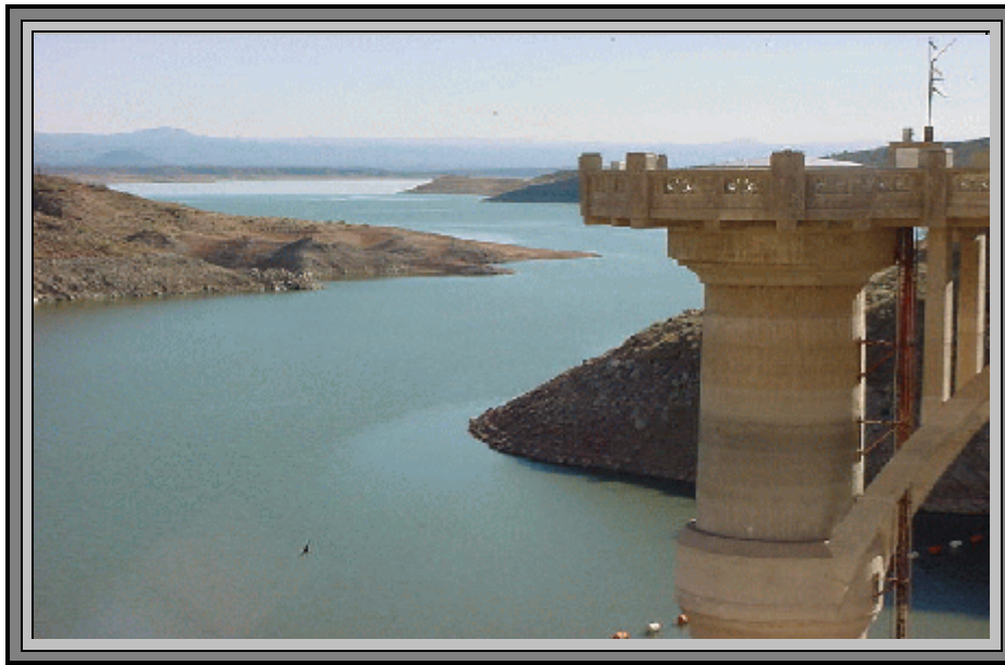
Figure 31. Coolidge Dam, constructed in 1928, impounds the Gila River upriver of the LSP and creates San Carlos Reservoir. Water is stored here for power generation and irrigation in San Carlos Irrigation Project lands near the Coolidge/Casa Grande area. The USGS collects water quality samples from the river near Calva upgradient of the reservoir. All ready highly mineralized especially during low flows 10 , evaporation from the reservoir adds to the salinity concentrations 32 . This surface water recharges the floodplain aquifer in portions of the LSP. Water is released from San Carlos Reservoir into the Gila River according to regulations contained in the Gila Decree of 1936 for San Carlos Project lands 10 .
