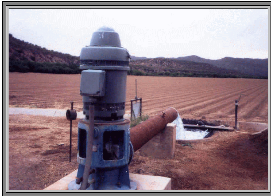
Figure 9. Powered by a turbine pump, a well draws groundwater from the floodplain aquifer for delivery to a field planted with cotton seed. Furrow irrigation systems are used to distribute water to scattered fields of cotton grown between the towns of Mammoth and Kearny. Recently, some fields are being replanted to riparian vegetation in an attempt to replace willow flycatcher habitat lost during the recent expansion of Roosevelt Dam and Lake. The pictured field is located near the confluence of the San Pedro River and Aravaipa Creek.
