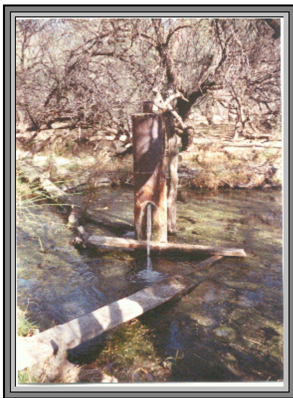
Figure 10. An artesian well creates a riparian area amidst a mesquite bosque near the San Pedro River just south of the town of Mammoth. Tapping the confined basin-fill aquifer, this 1485 foot deep well drilled in 1934 spills water out of the casing at a hot 38.6 degrees Celsius. Groundwater chemistry—very soft with elevated levels of pH and fluoride—is suggestive of a chemically-closed system.
