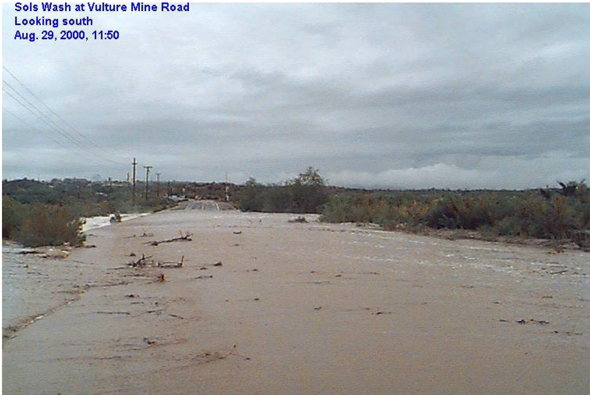
Sols Wash at Vulture Mine Road, view to south, Aug. 29, 2000 at 11:50
