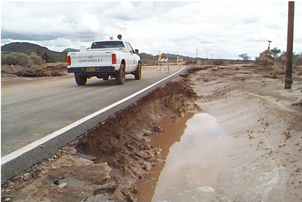
Centennial Wash @ Harquahala Valley Road - 10/23/2000
