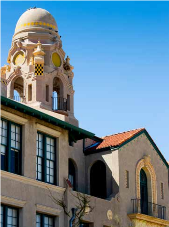
The Curley School Artisan Housing Center, located in a historic public school in Ajo, Arizona.
