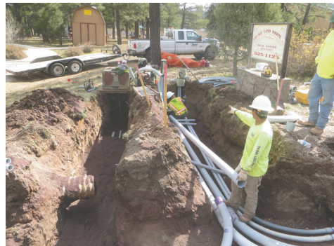
Kachina Trail Reconstruction Project
