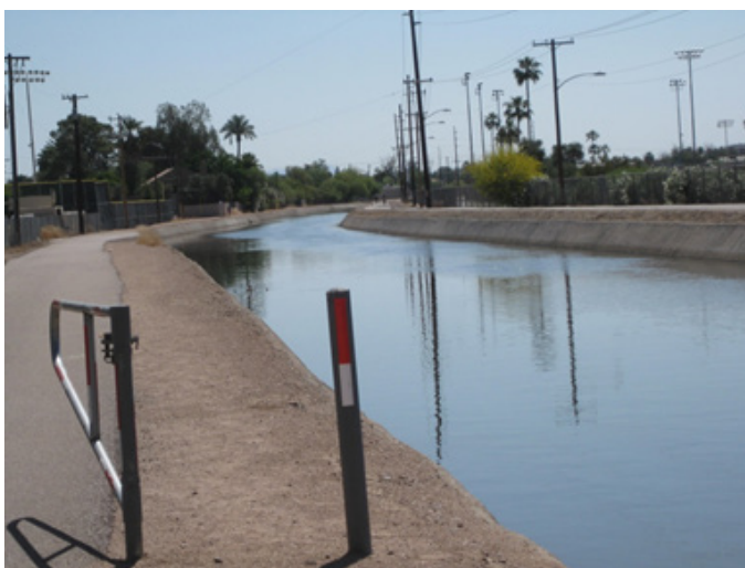
Figure 3. Paved pathways along the Canal
