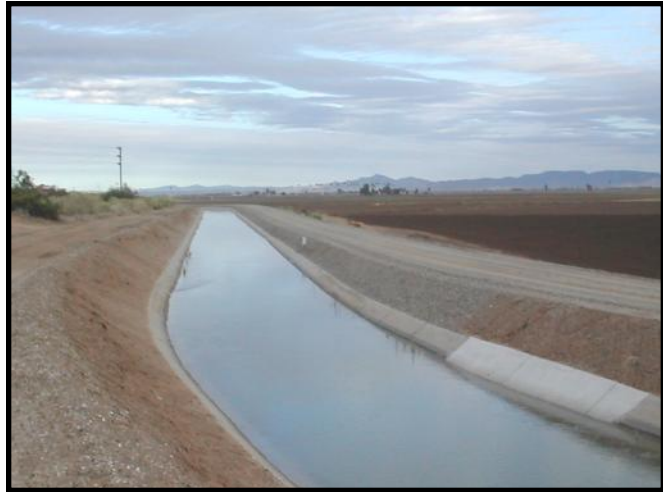
South Gila Valley Canal
