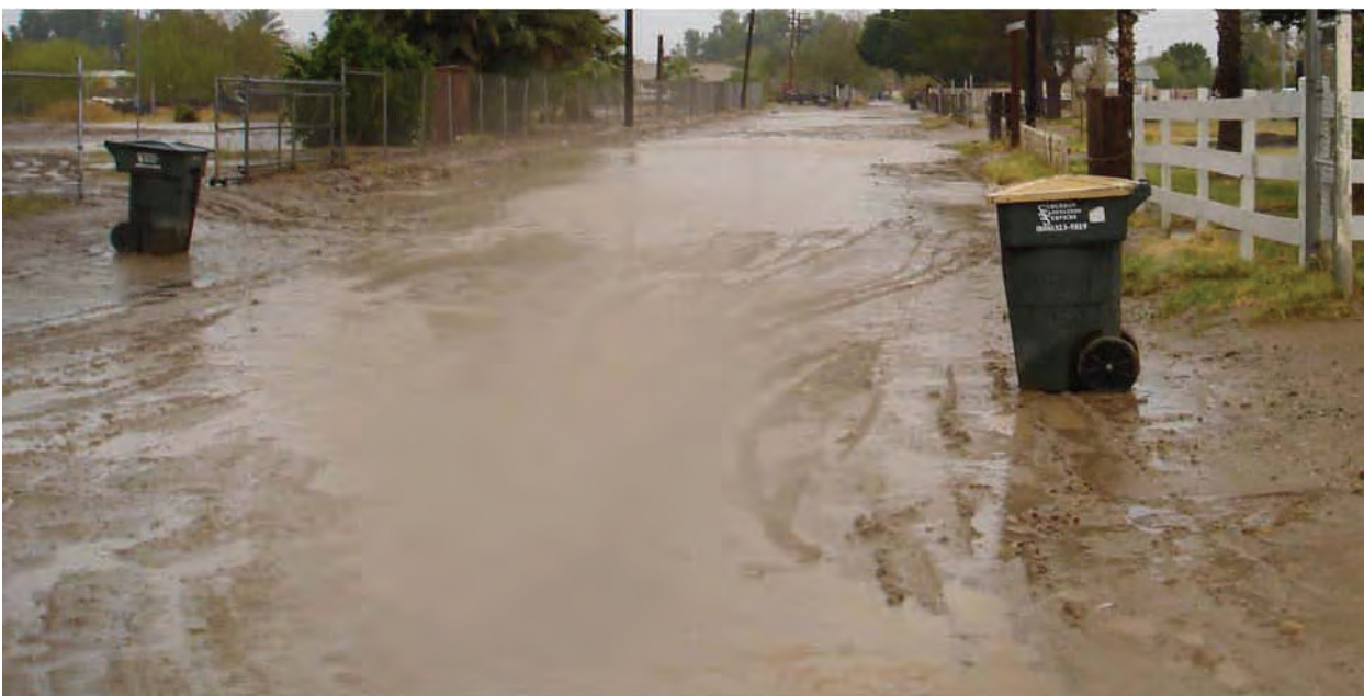
An unpaved and unmaintained street after a heavy rainfall
