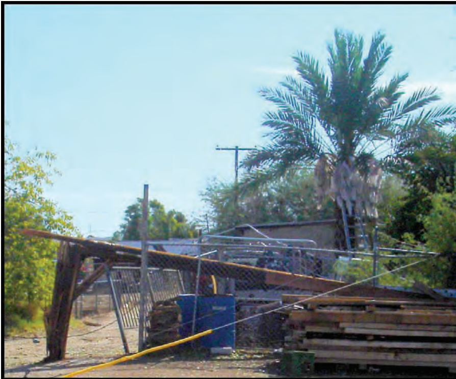
Power pole that has been broken by a thunderstorm
